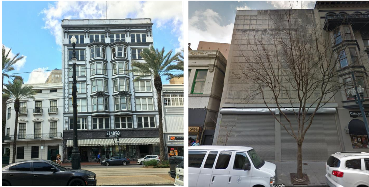
Figure 42: 826 Canal Street (left), 120 Baronne Street (right)
