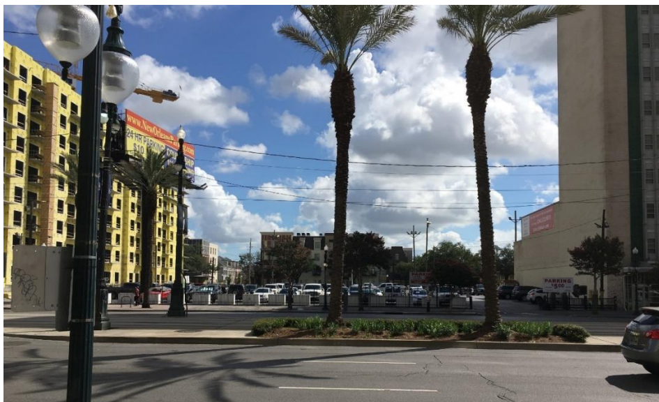
Figure 82: Surface parking lot located at 1539 Canal Street
