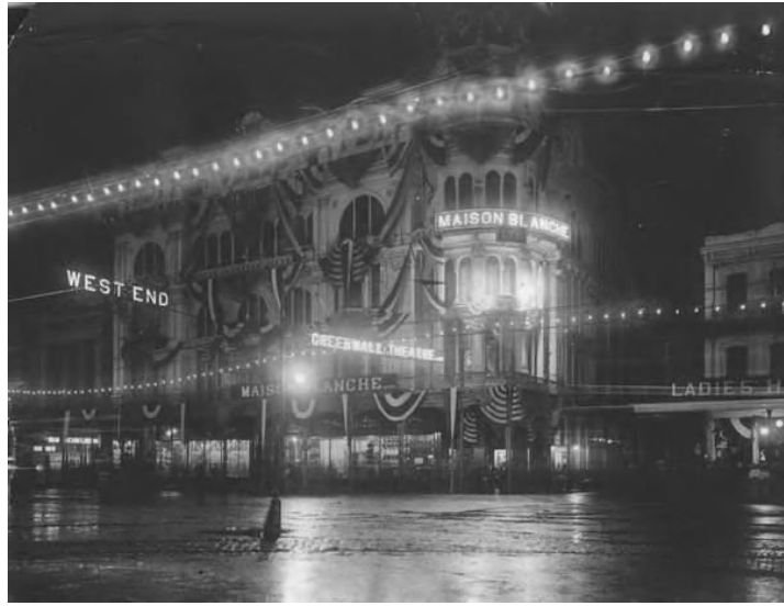
Figure 3 & Figure 4: Original Maison Blanche building (top) and its replacement (bottom)
