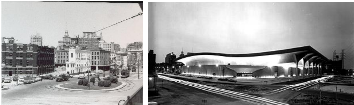
Figure 23 & Figure 24: Historic structures at foot of Canal Street (left) 66 and Rivergate Exhibition Hall (right) 67
