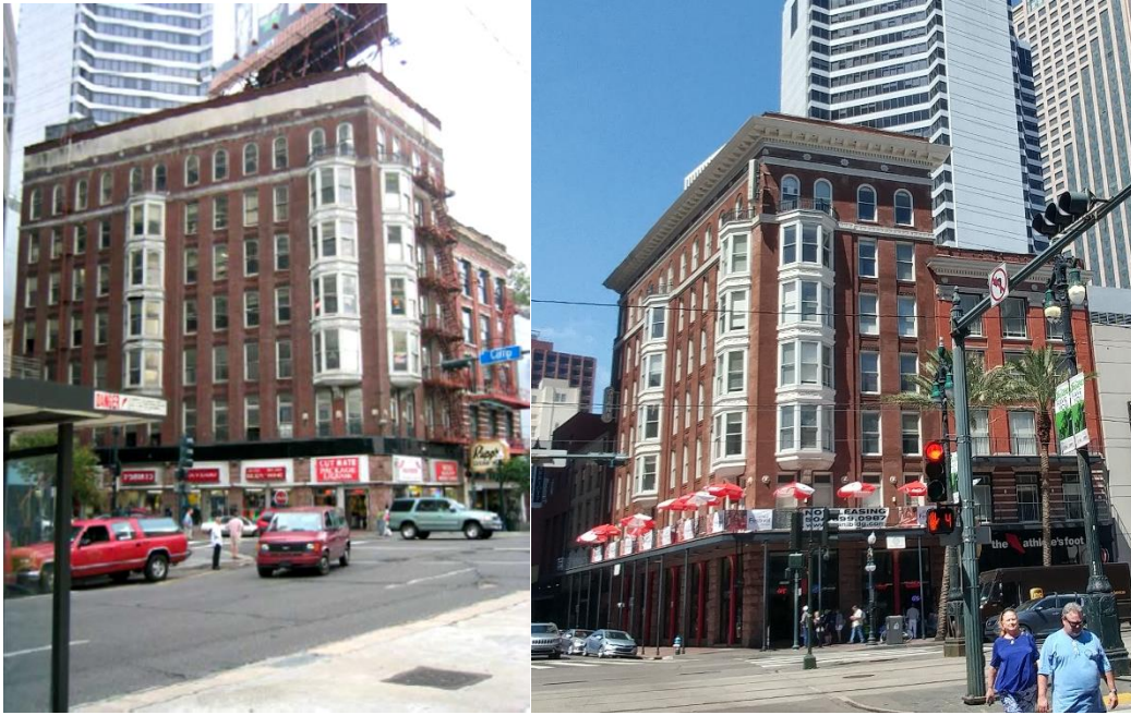
Figure 71 & Figure 72: Giani Building pre-renovation (left) and post-renovation (right)
