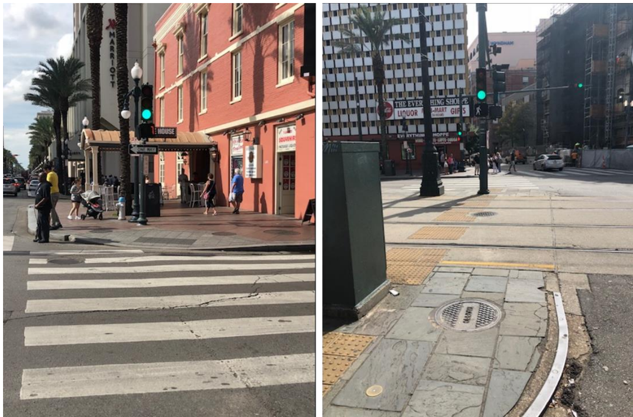
Figure 64: Pedestrian Improvements along Canal Street
