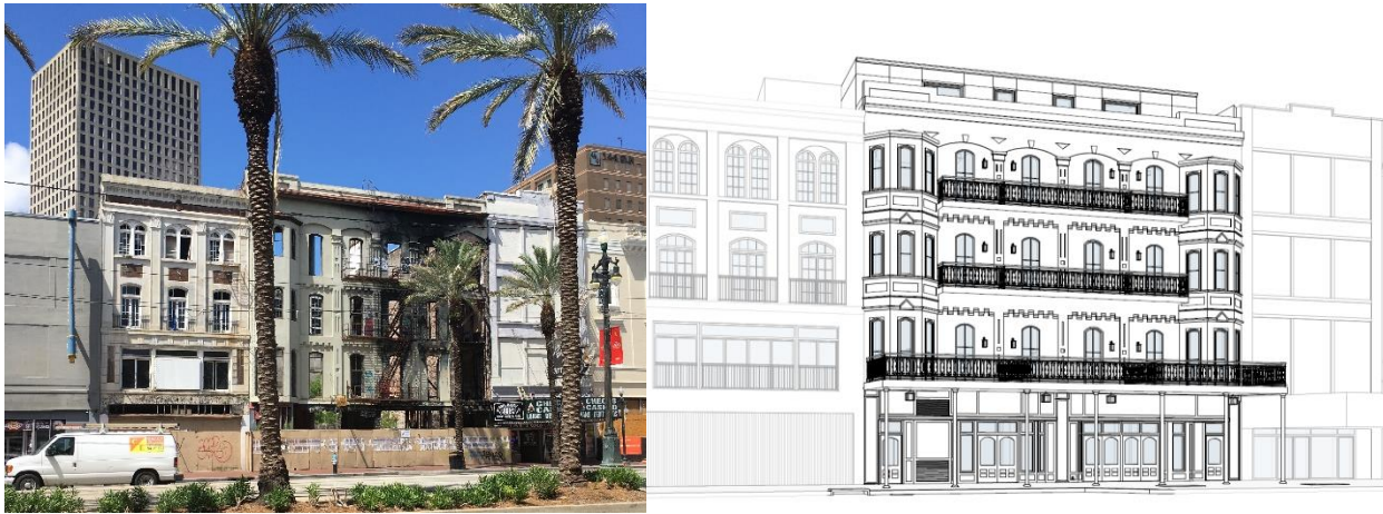
Figure 47 & Figure 48: 1016 Canal Street after fire (left) & Elevation of Proposed Construction (right)
