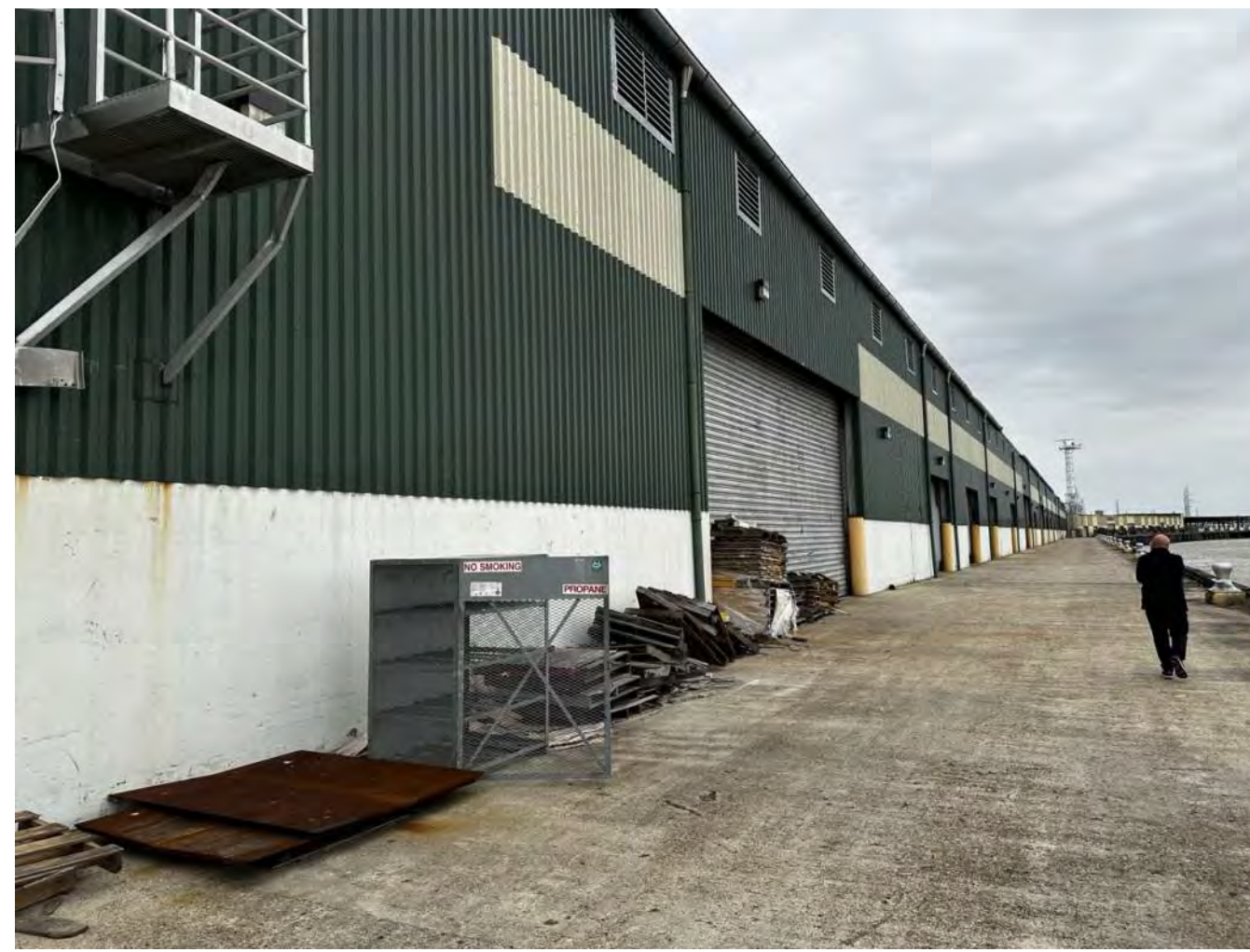
14 EXISTING CONDITION IMAGE 1.21A | 1/64" = 1'-0"
