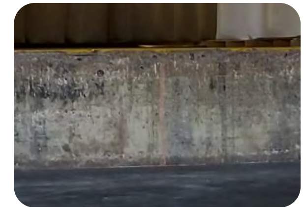
EXISTING CONCRETE WALLS
