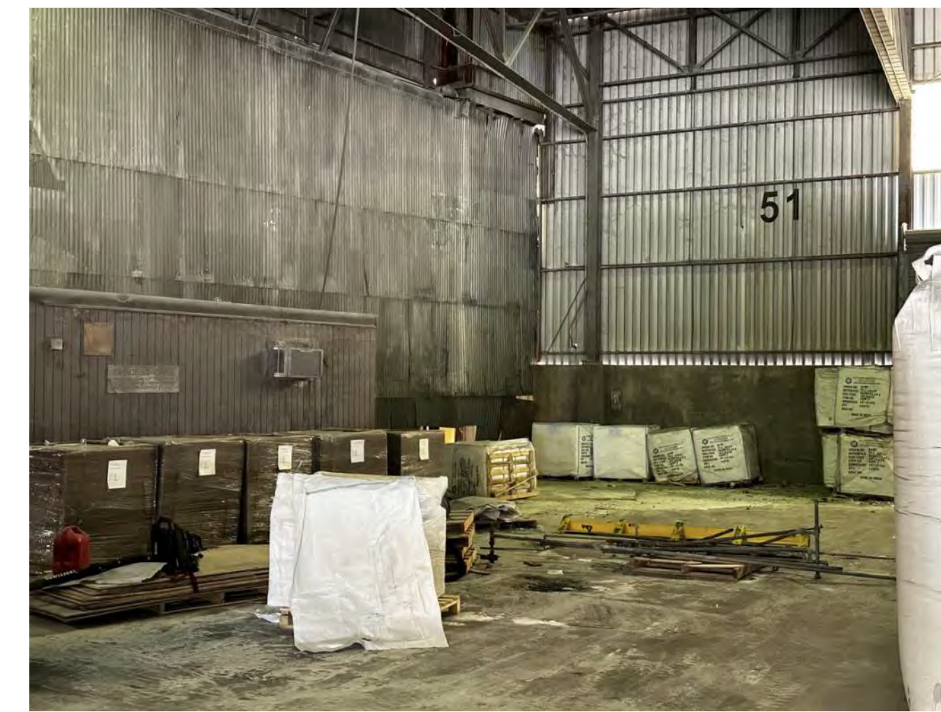
06 EXISTING CONDITION IMAGE 1.21C | 1/64" = 1'-0"
