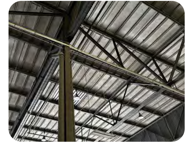
EXISTING STEEL TRUSSES
