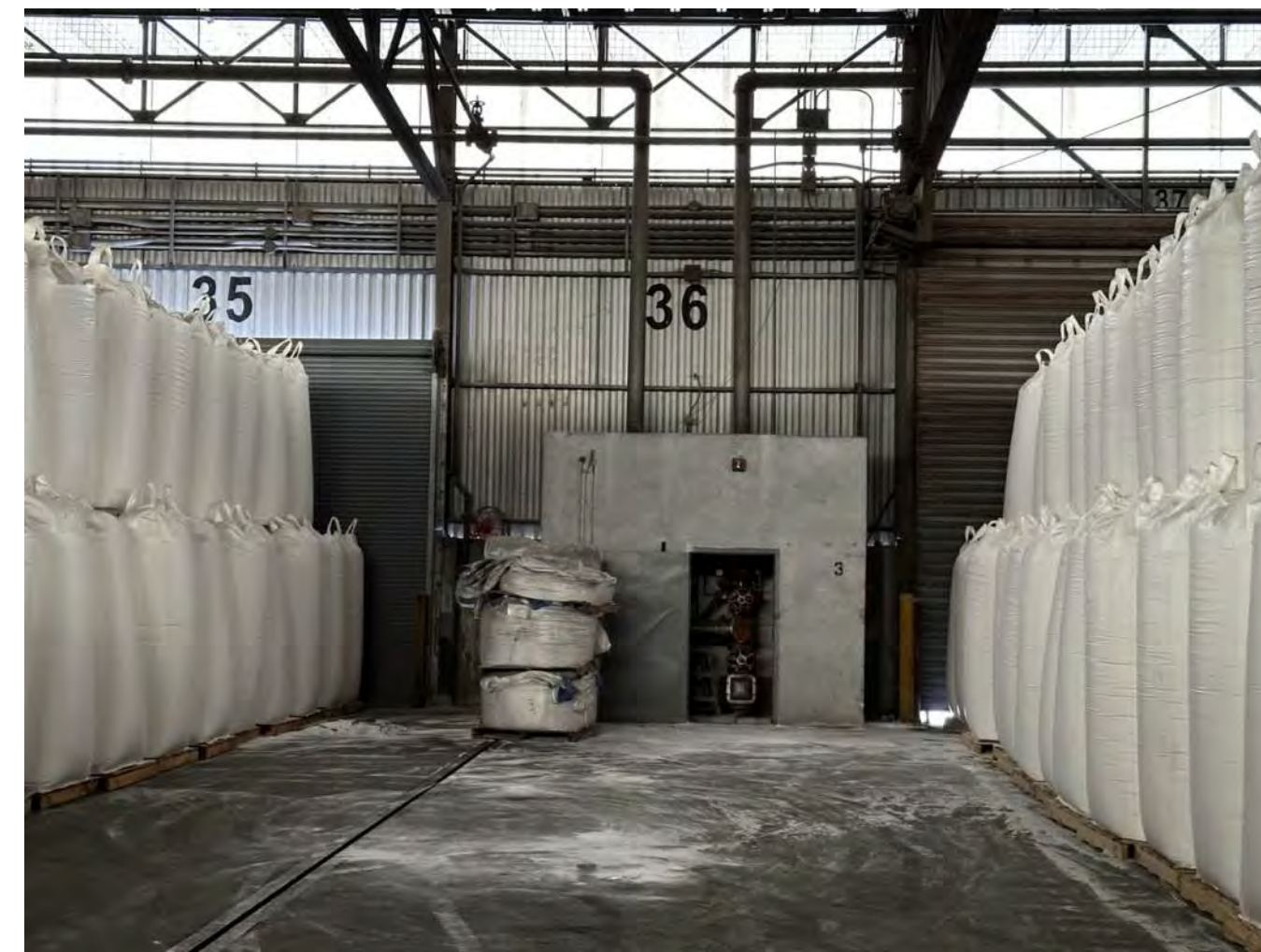
09 EXISTING CONDITION IMAGE 1.21C | 1/64" = 1'-0"
