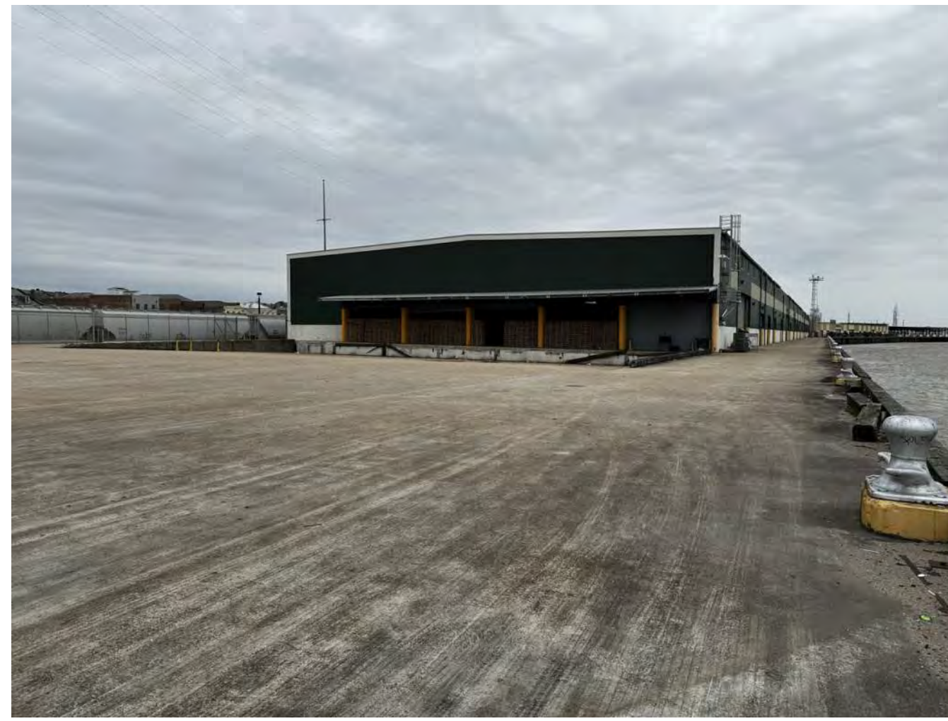
15 EXISTING CONDITION IMAGE 1.21A | 1/64" = 1'-0"
