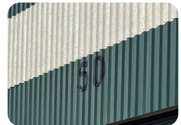
EXISTING METAL PANELS
