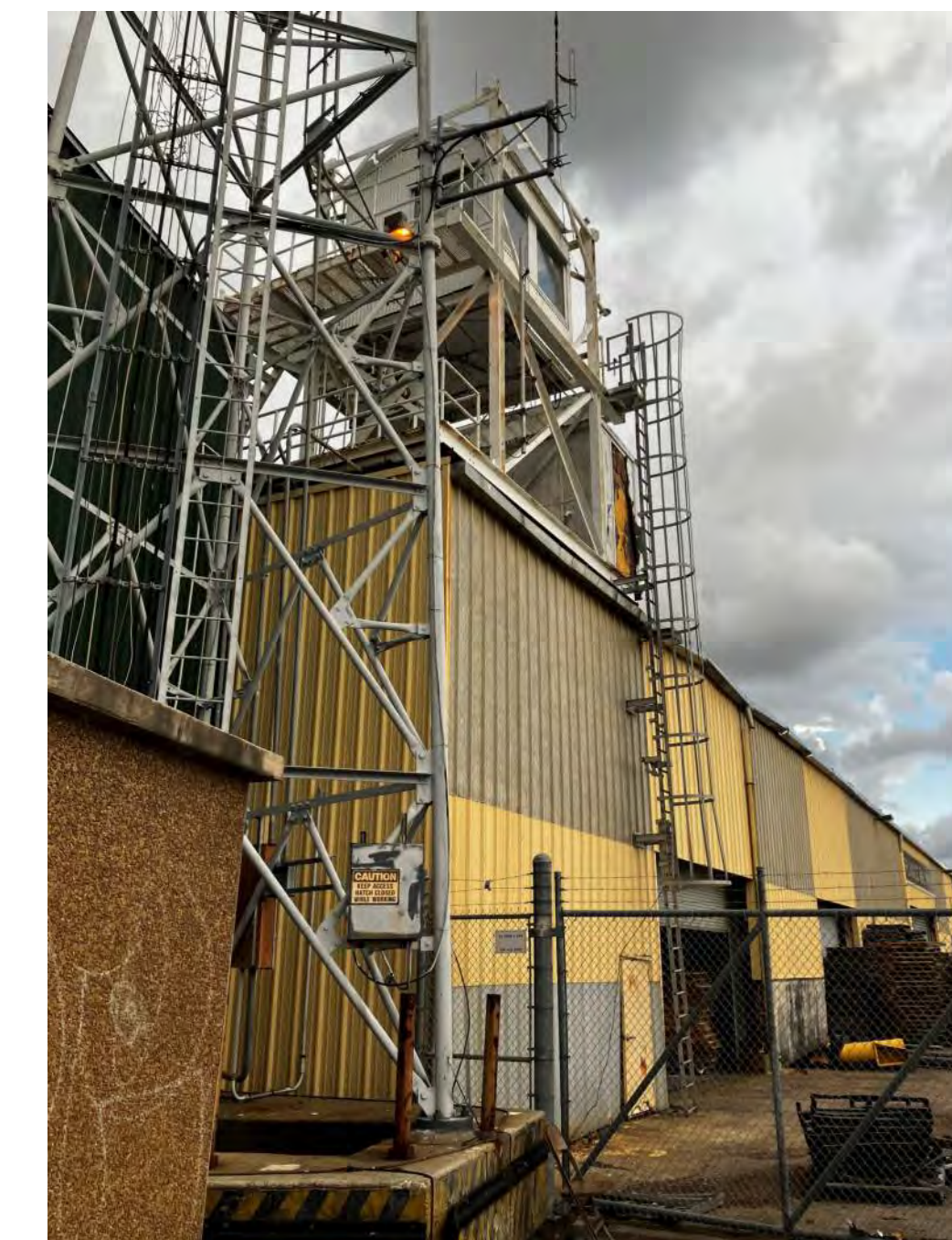
01 EXISTING CONDITION IMAGE 1.21C | 1/64" = 1'-0"
