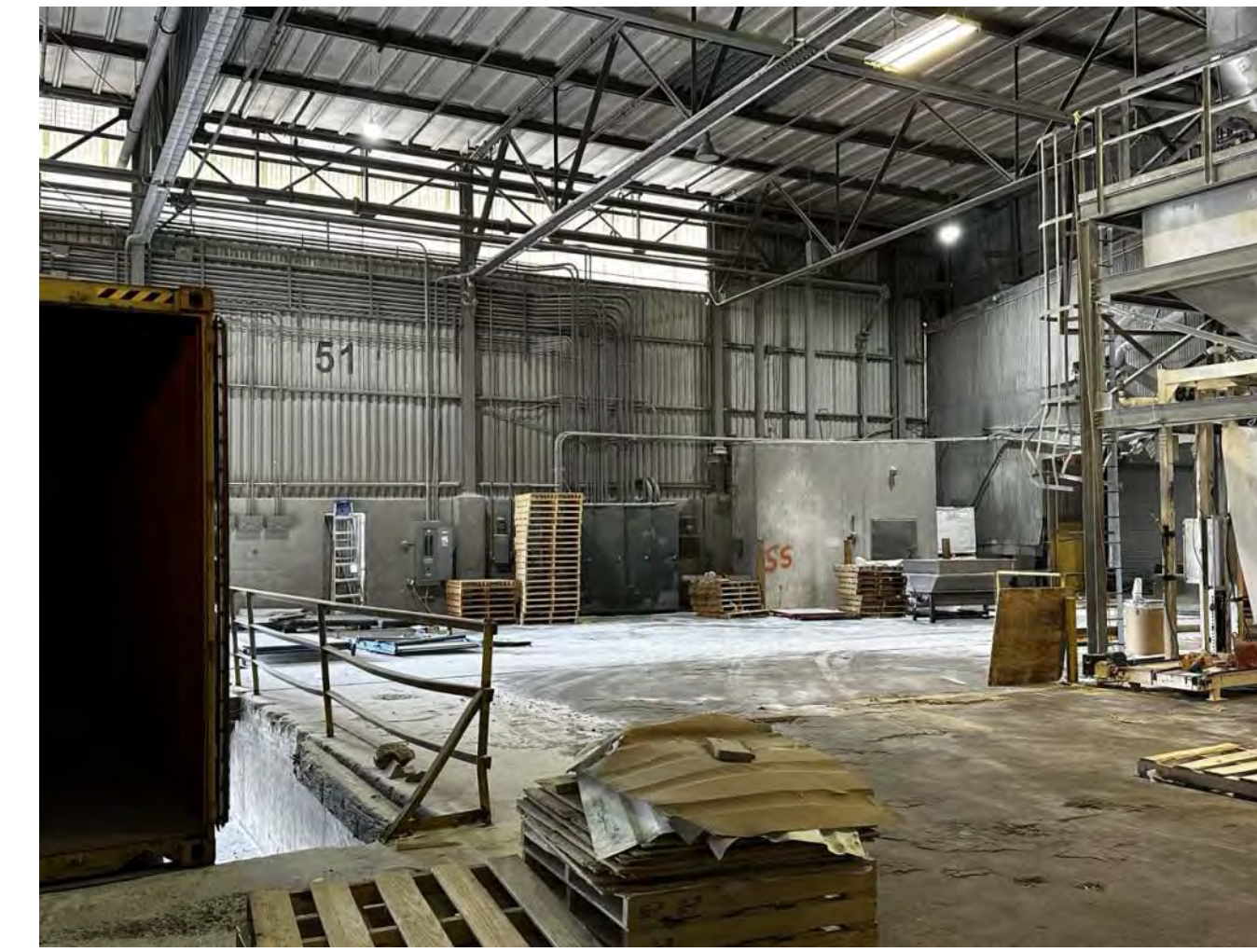
07 EXISTING CONDITION IMAGE 1.21C | 1/64" = 1'-0"
