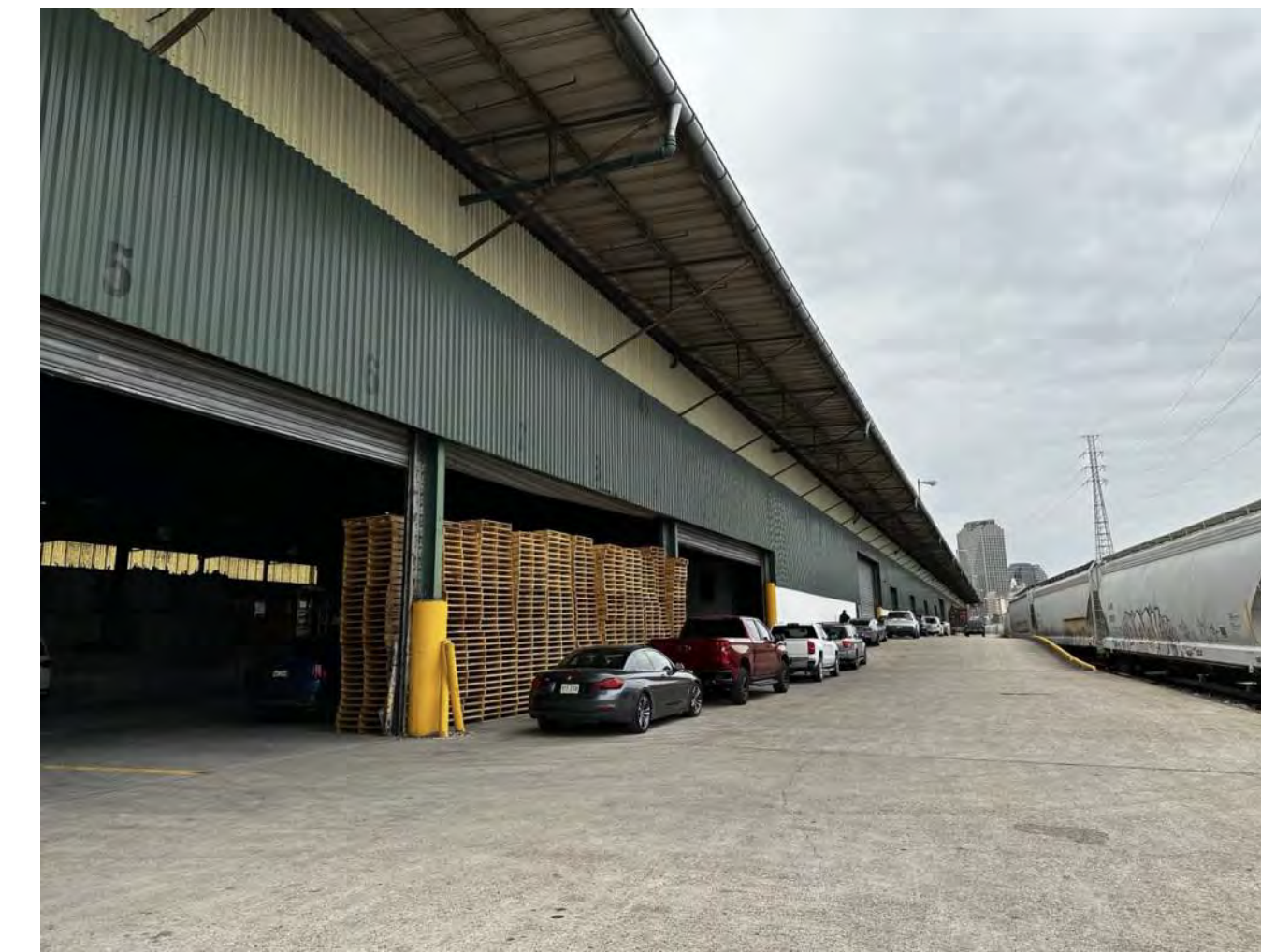
05 EXISTING CONDITION IMAGE 1.21C | 1/64" = 1'-0"
