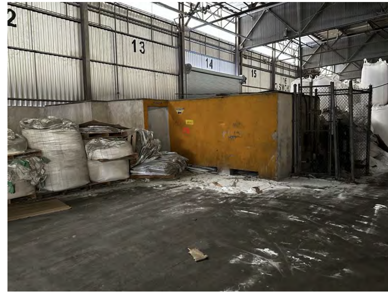
11 EXISTING CONDITION IMAGE 1.21A | 1/64" = 1'-0"
