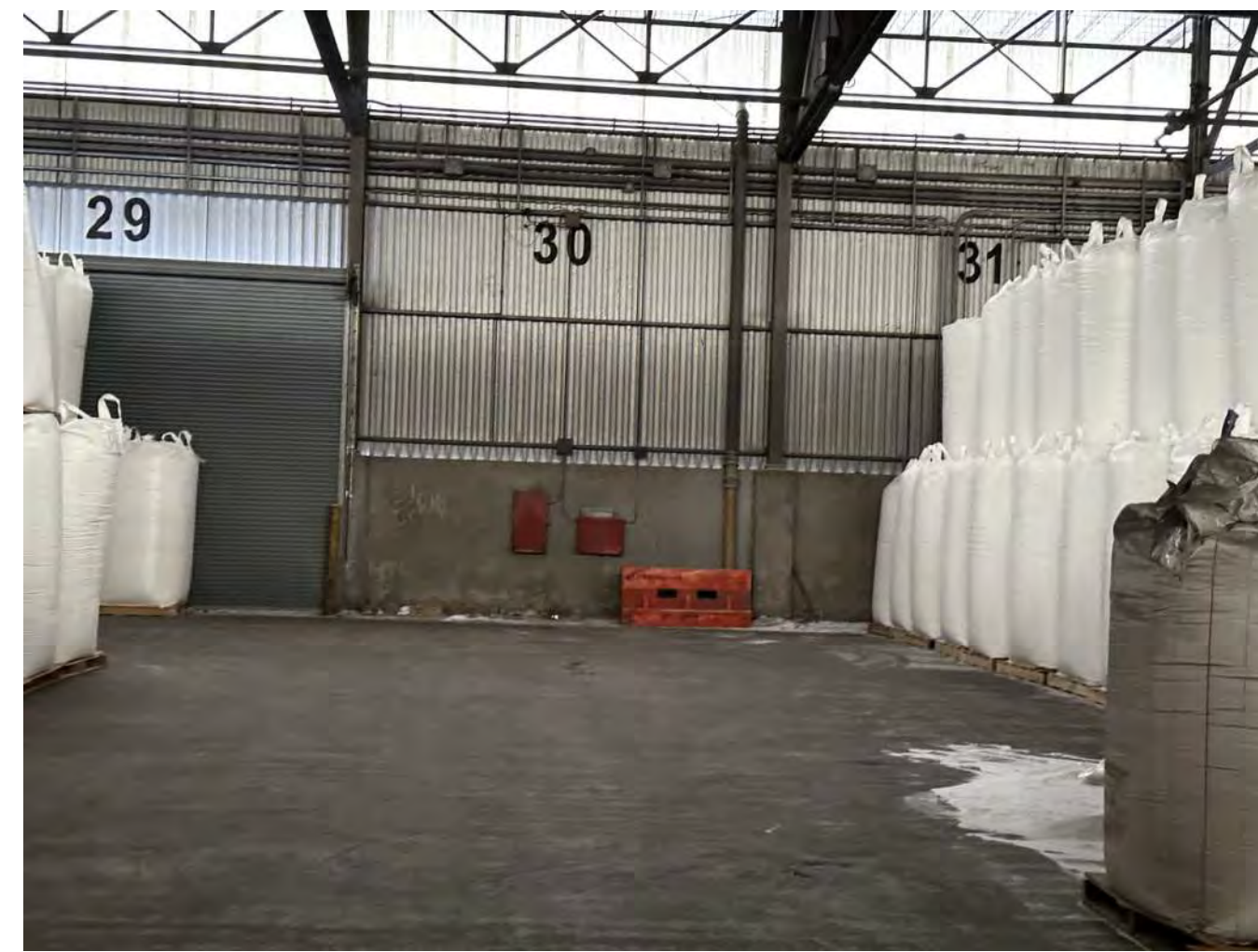
10 EXISTING CONDITION IMAGE 1.21B | 1/64" = 1'-0"
