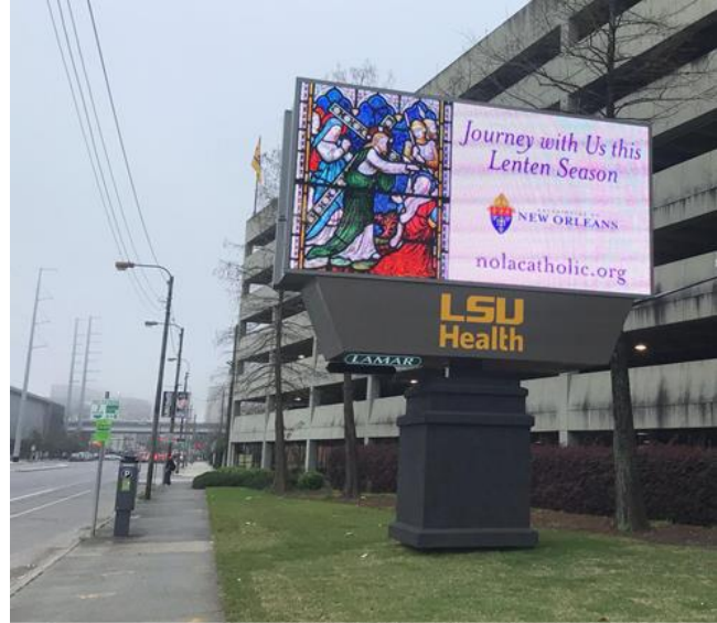
Figure 10. Example of a billboard with digital display with a monument-type support structure.
