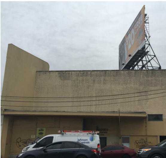
Figure 11. Example of a billboard with an A-frame support structure.
