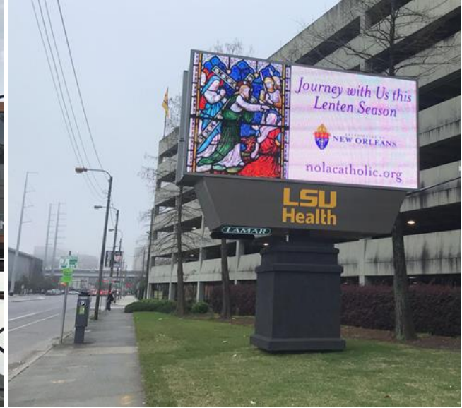
Figure 10. Example of a billboard with digital display with a monument-type support structure.
