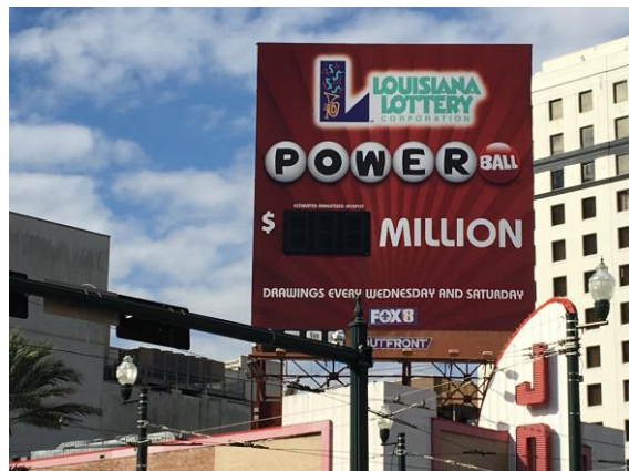
Figure 2. Example of a billboard, or off-premises advertising sign, mounted to the roof of the Joy Theatre on Canal Street.
