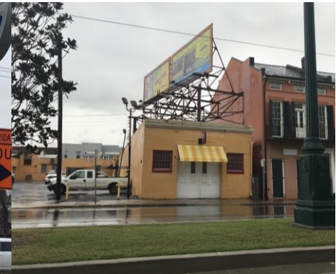
Figure 26. Decked billboards roof-mounted on building in the Vieux Carre.
