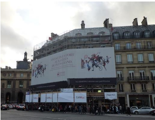
Figure 19. Advertising on building scaffolding in Paris. Photo: Didier Rykner
