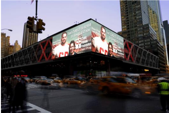
Figure 43. Wall mounted billboard incorporated into facade of new public building
