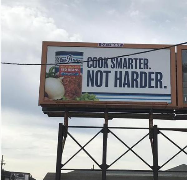
Figure 9. Example of a billboard with static display and an I-beam support structure.
