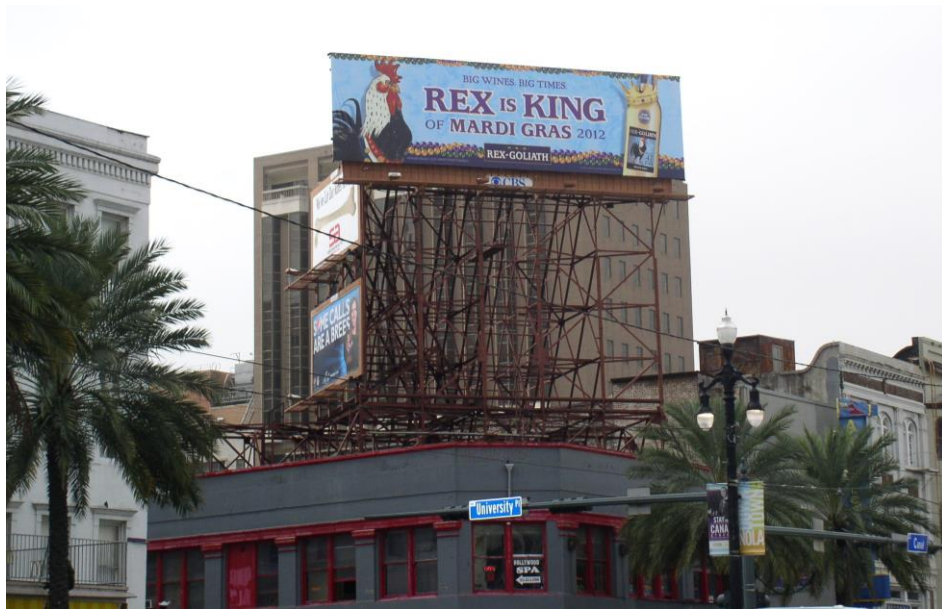
Figure 29. Roof-mounted billboard on Canal Street
