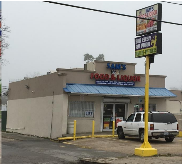
Figure 35. 2019 photo of renovated structure showing removal of billboards and other excessive signage and façade improvements.
