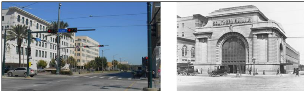
Figure 66 & Figure 67: Southern Railway Station Site Present (left) and Prior to Demolition (right)
