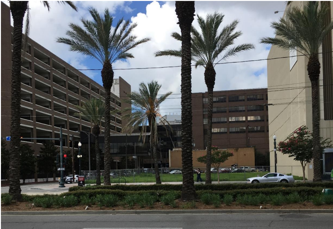
Figure 80: Vacant lots located at 1400 Canal Street
