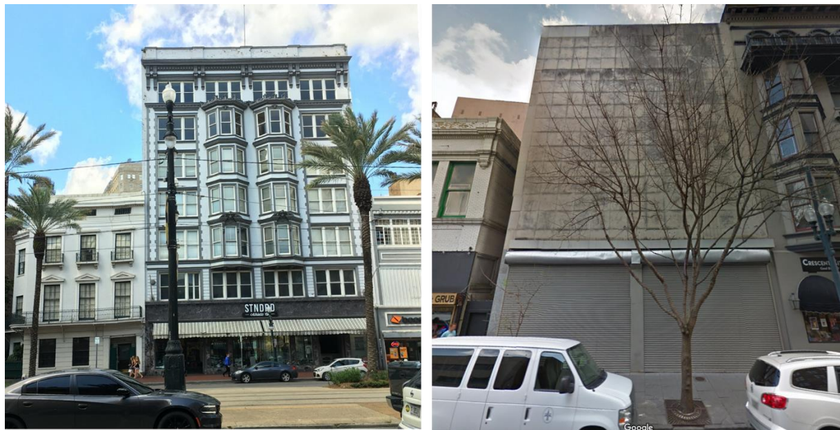
Figure 42: 826 Canal Street (left), 120 Baronne Street (right)
