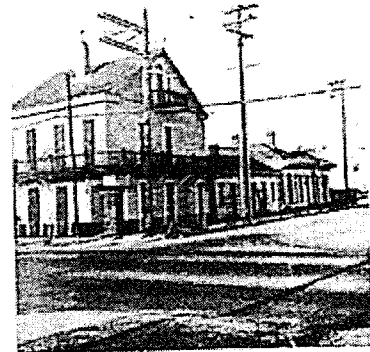
A complex of newly restored buildings on Elysian Fields Avenue at Royal St.
