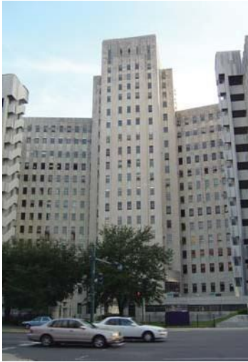
The Medical Center of Louisiana at New Orleans (MCLNO/Charity Hospital) was the region’s primary safety-net provider of care for residents without insurance before Hurricane Katrina.
