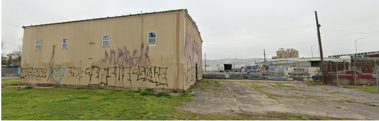
Figure 2. Vacant Warehouse and Slab on Subject Site (Source: Google Maps)
