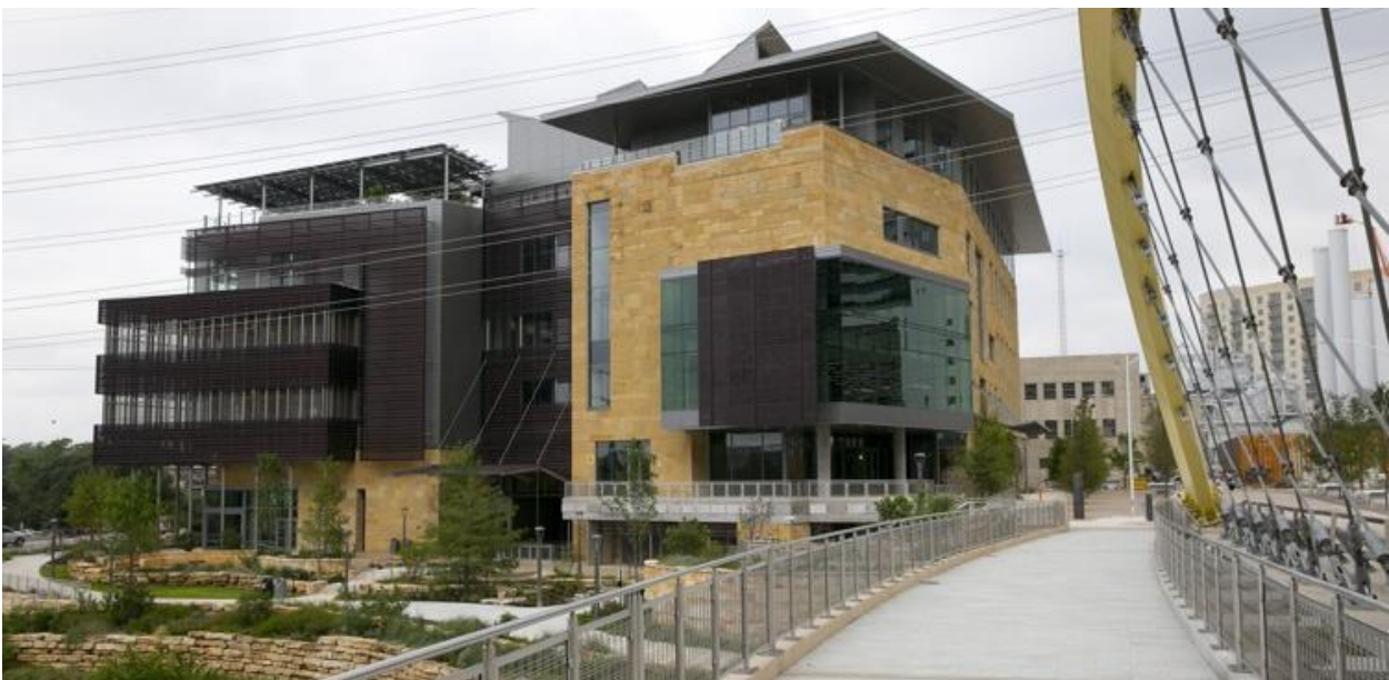
Figure 7. Austin Central Library nearing completion in 2017. https://www.mystatesman.com/news/local/austin-new-central-library-due-open-oct/DWck9o6fhQ7E4YWbt5Jq7N/
