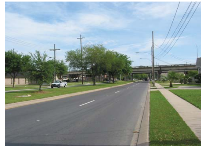
Transcontinental at the I-10 underpass
