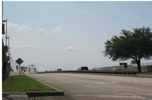
Hayne Blvd. with Sen. Ted Hickey Bridge in background
