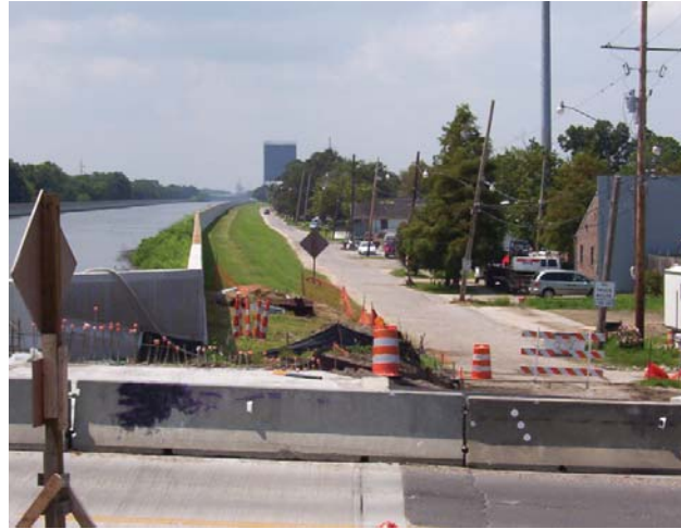
Intersection of Orpheum St. and Hammond Hwy (looking river bound)
