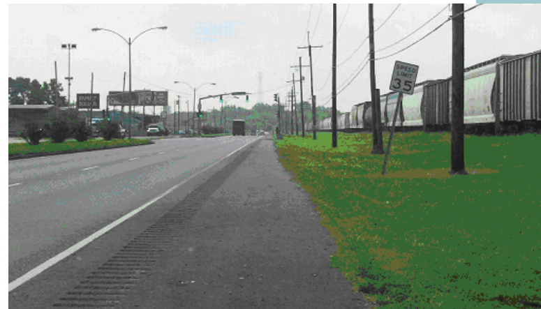
Rumble strips on LA 46 on newly repaved surface
