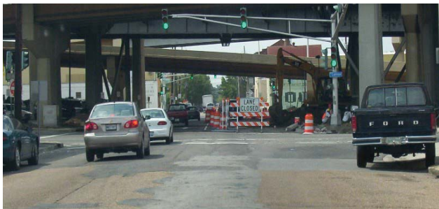
Magazine Street on-way westbound at Pontchartrain Expressway (ramp modifications under construction)
