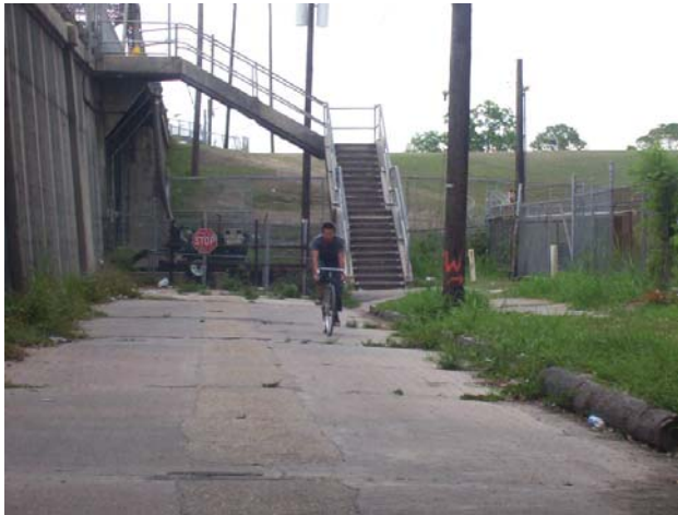
St. Claude Service Road to pedestrian bridge
