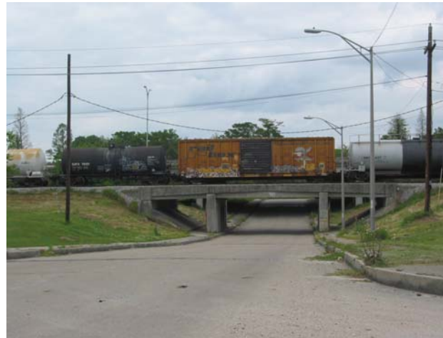
I-10 and railroad underpass in City Park
