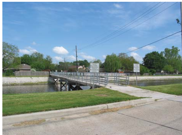
Pedestrian/Bike bridge over Elmwood Canal
