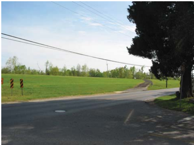
Central Ave. and Jefferson Hwy. Levee path access via gravel ramp.
