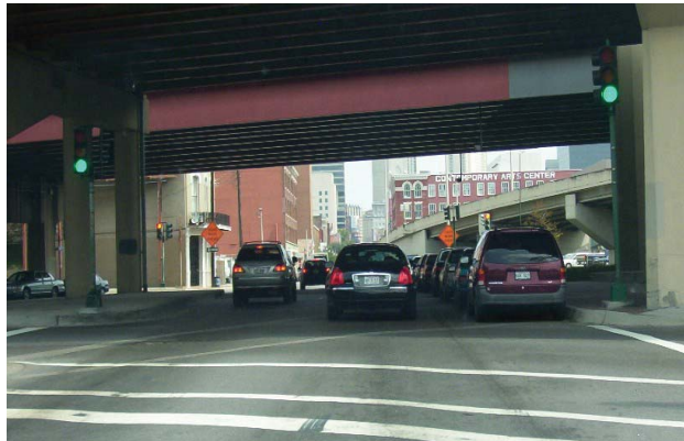
Camp St. one-way eastbound at Pontchartrain Expressway with on-street parking underunderpass
