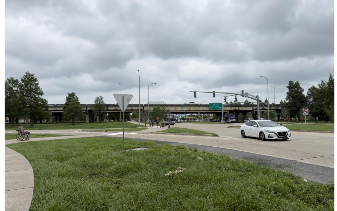
Segment D - Bullard Ave Interchange Conditions After
