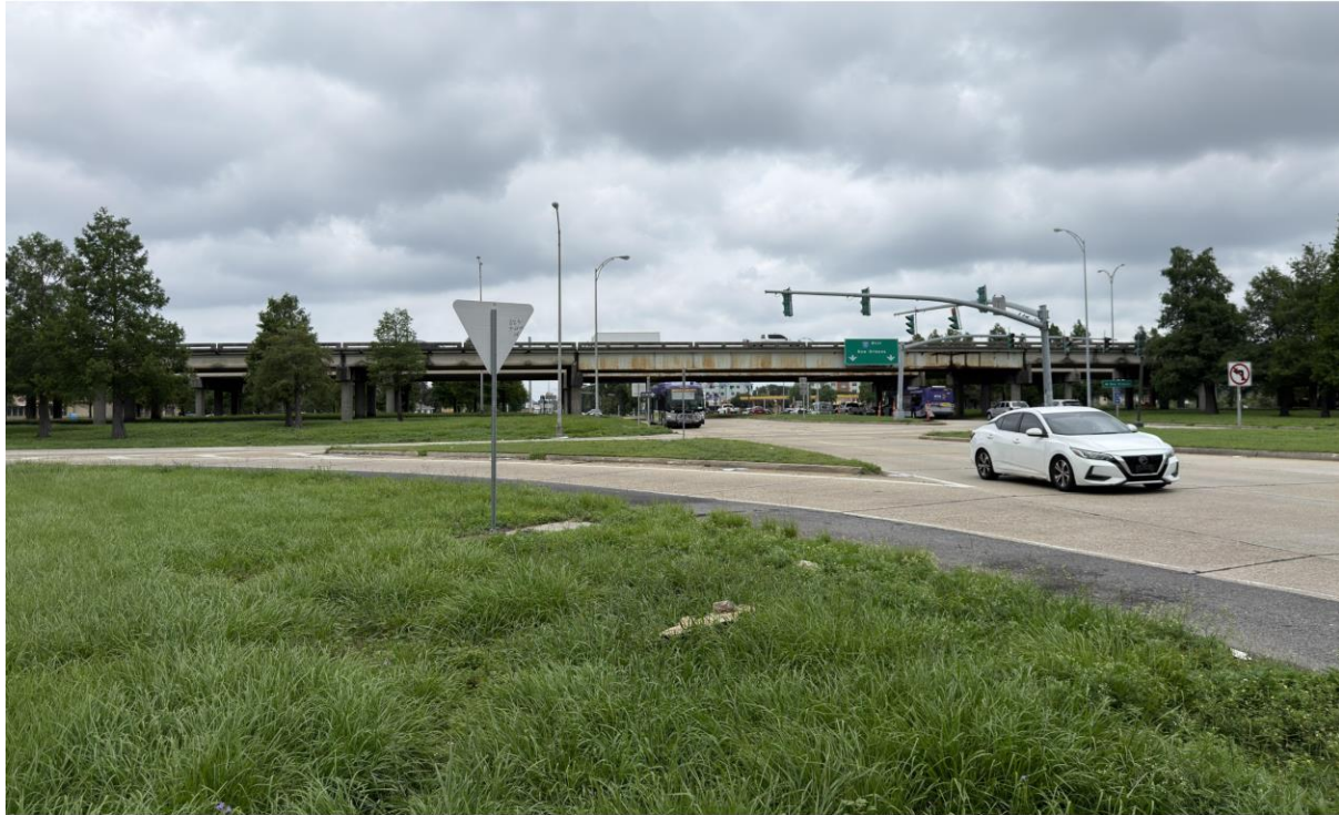
Segment D - Bullard Ave Interchange Conditions Before
