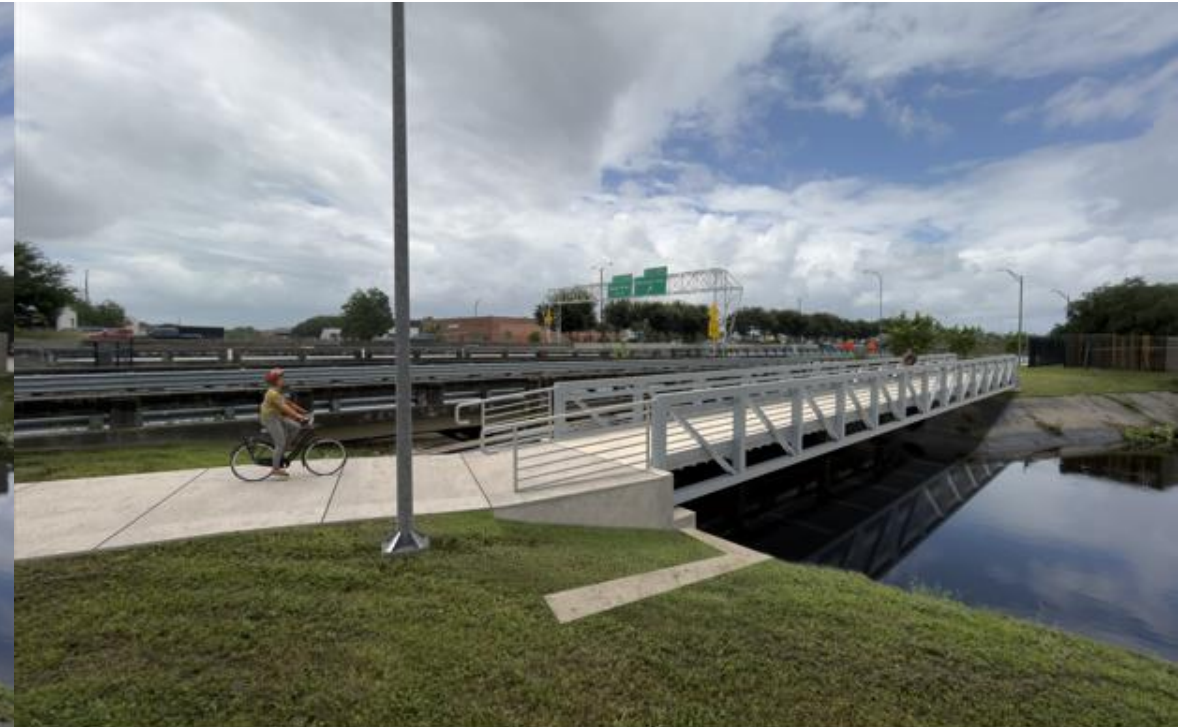
Segment D1 - N I-10 Service Rd. Bullard Ave to Shadowlawn Dr Conditions After
