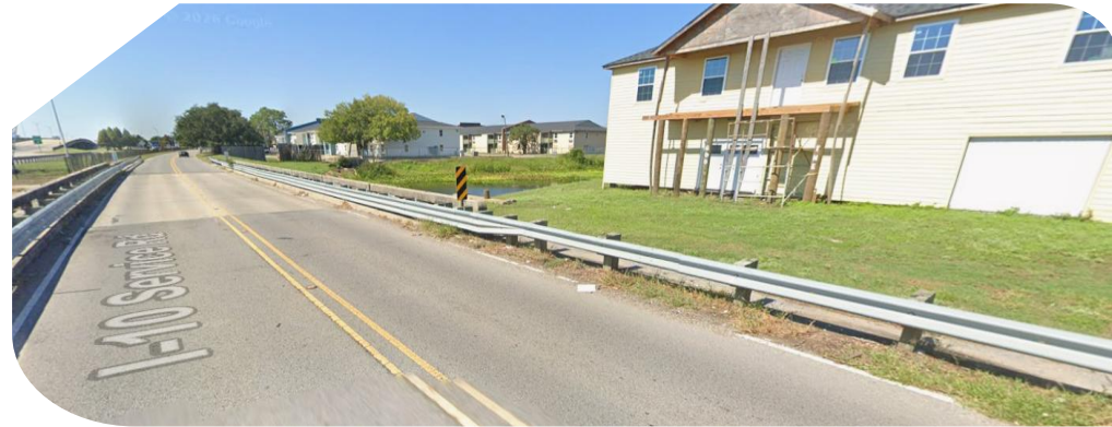
Jahncke Canal at North Service Road
