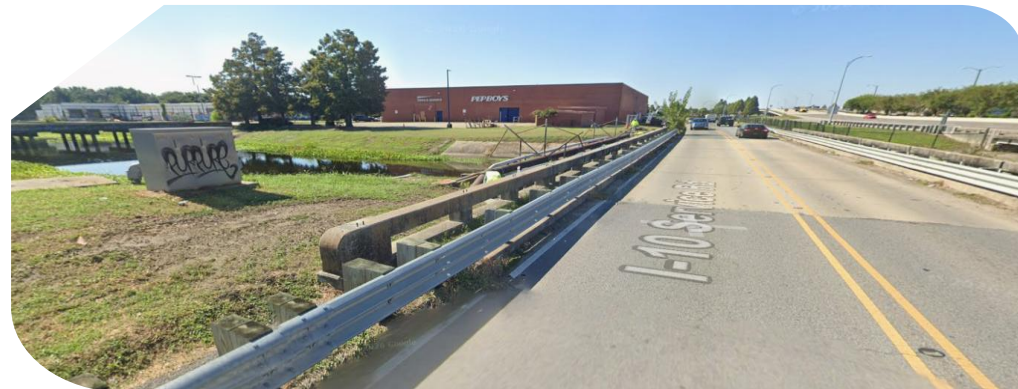
Jahncke Canal at South Service Road
