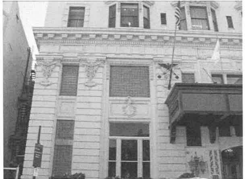
Beaux Arts detailing of shields, floral design, elaborate cornice and rusticated walls.
