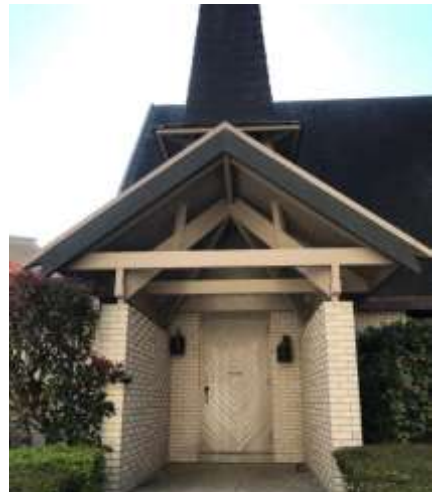
Figure 30. Entry vestibule, 1772 Prytania St., 2019
