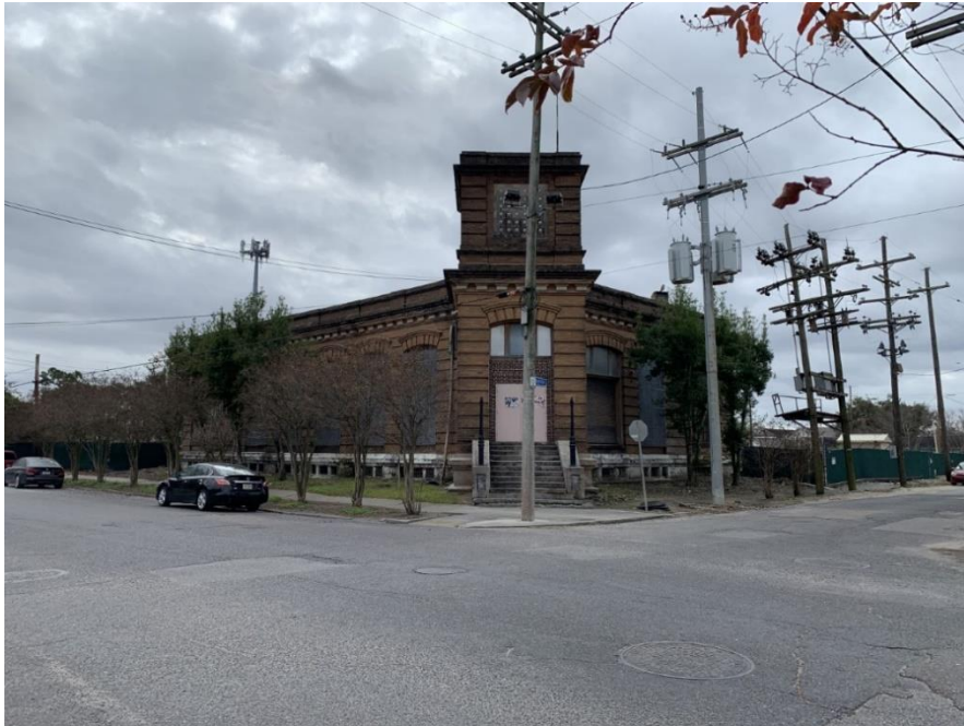
Figure 11. Valence Street Substation, 2021
