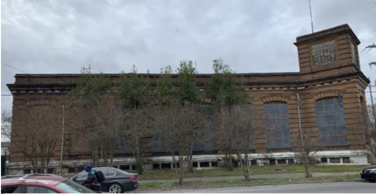
Figure 13. Valence Street Substation, 2021
