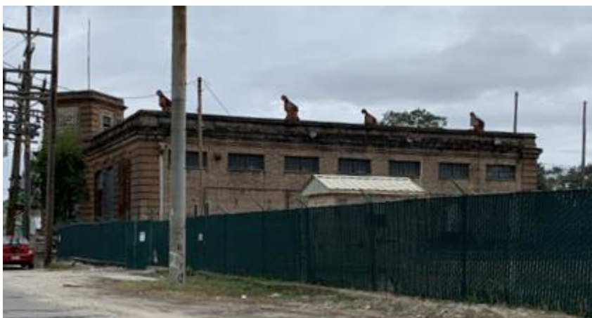
Figure 12. Valence Street Substation, 2021
