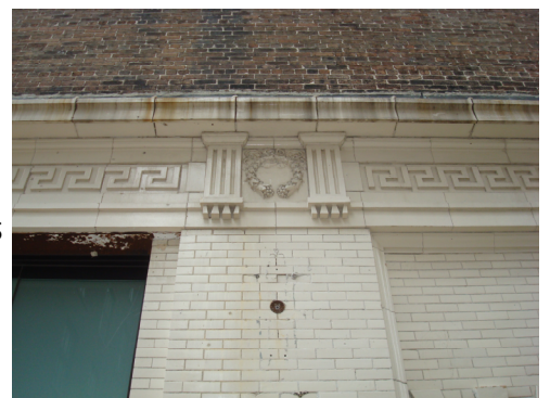
Figure 10 below: Detail of terra cotta ornament on façade. September 9, 2008.
