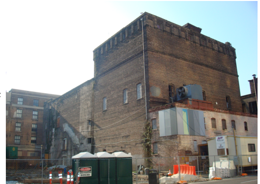
Figure 12: Rear and north elevations of the theater. September 9, 2008.
