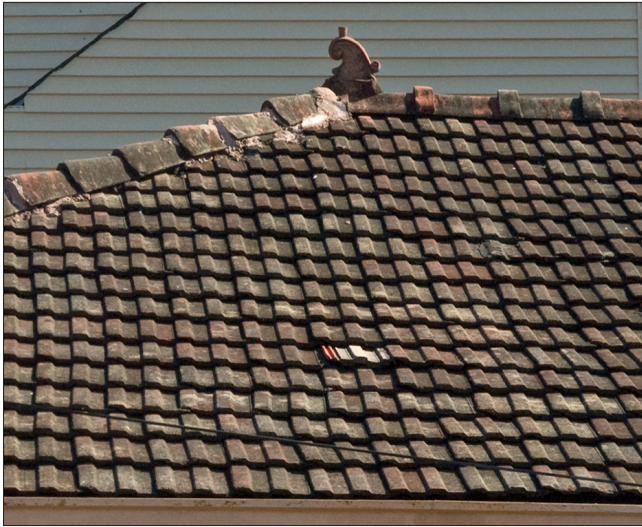
This concrete tile roof includes a finial and terra cotta ridge caps at the top of the main roof and along the roof hip.
