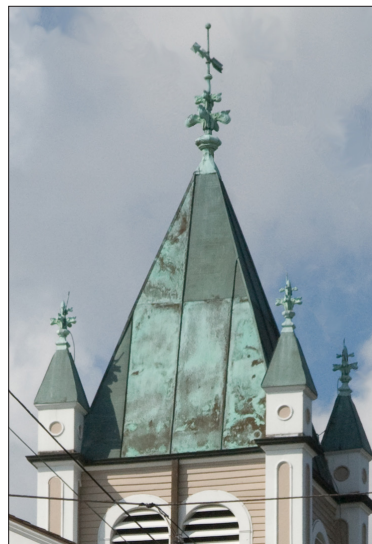
The top of this church tower includes a standing seam copper roof, copper finials and a weathervane. Copper roofing is known for its longevity with relatively little required maintenance.
