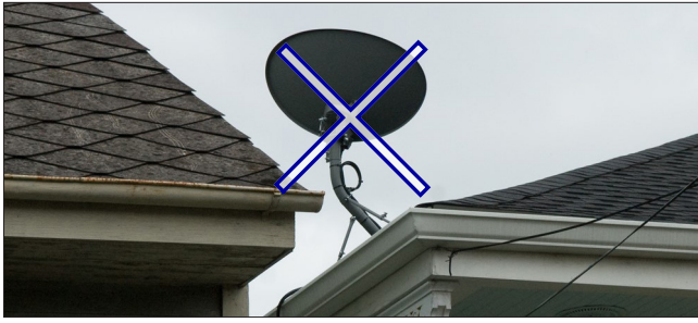
Satellite dishes should be installed towards the rear of the building so they are minimally visible from the street.
