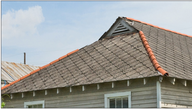
The asbestos shingle roof has terra cotta caps on the ridge and hips and a triangular louvered vent at the front gable. The ridge caps and louvered vents should be retained. Gutter installation is recommended.
