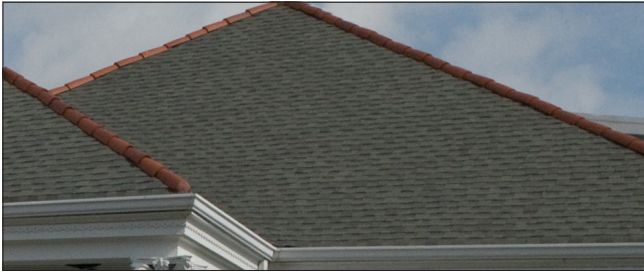
This dimensional asphalt shingle hipped roof features ridge tiles at the hips and a perimeter gutter.
