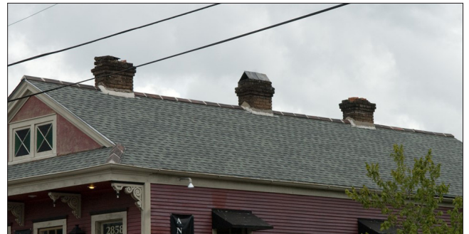
This row of three chimneys suggests the division of rooms on the interior of the building. The central chimney includes an inverted "V" cap and English V ridge tiles with mortared joints marking the top of the roof.
