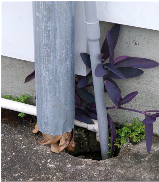
The downspout is clearly clogged with leaves and is discharging onto the sidewalk instead of into the drain. It is likely that the clogged downspout will overflow onto the building walls.
