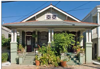
One-story homes are common in the District
