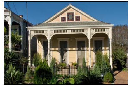
Cast iron fencing still edges the small front yards of many homes
