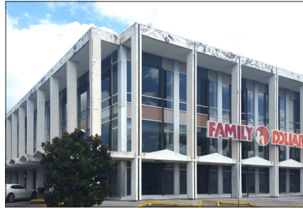
Many of the commercial buildings were constructed in the 1950s.
