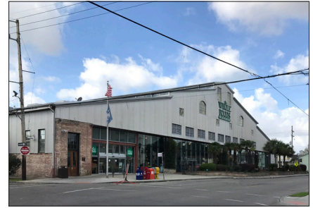
Many commercial buildings are concentrated along Magazine Street.
