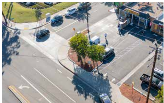
FIGURE 11 Access Management An example of driveway narrowing and median access management strategies in Costa Mesa, CA.
