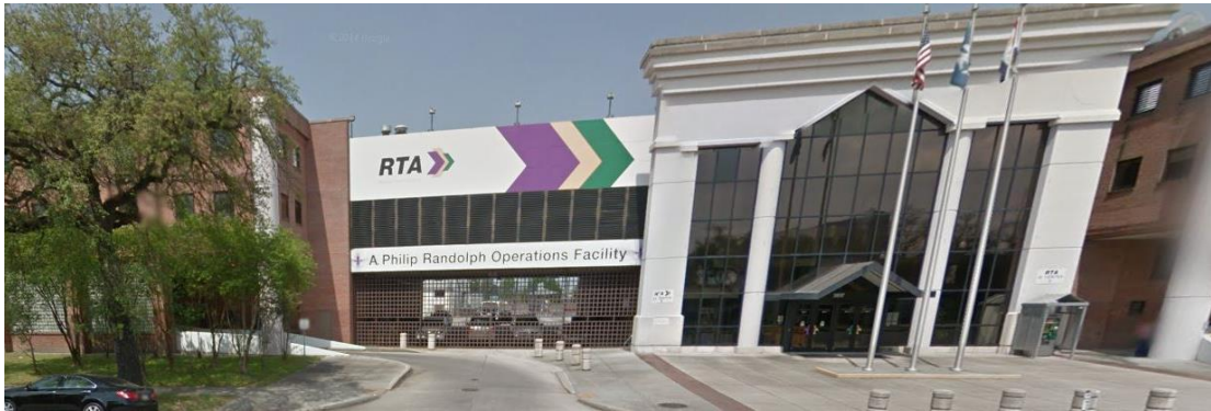
Figure 3: Front of RTA Building, Canal Street
