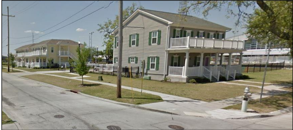
Figure 2: New residential units being constructed on the subject property
