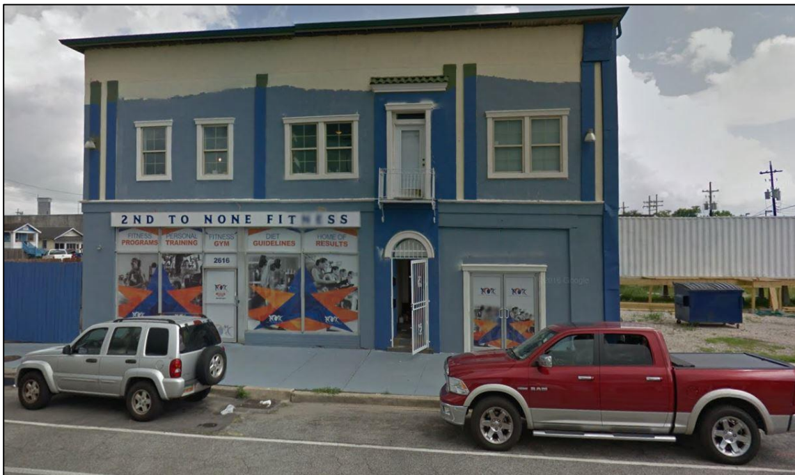
Figures 2 - 4: Pictures of existing structures in the Subject Area
