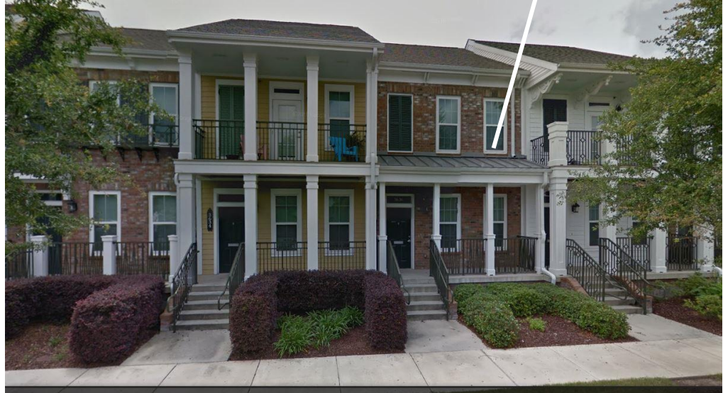
Figure 4: Columbia Parc, across Hamburg Street from Subject Property
