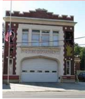
Upgraded police and fire stations will provide more reliable service in case of emergencies and can also serve as emergency shelters during storm events.
