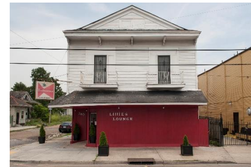
At-grade commercial buildings, typical in parts of the corridor, have increased flood risks.
