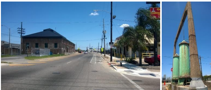
The pumping station at Broad St. and the Lafitte Greenway is a prominent landmark that could serve as an iconic focal point for public gathering, community space and water education.
