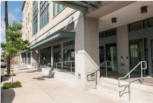
This example of new construction is a four story mixed-use infill development with an elevated ground floor.
