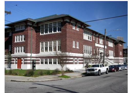
The recently renovated Myrtle Banks School building has offices on the upper floors and the Dryades Public Market on the main floor.
