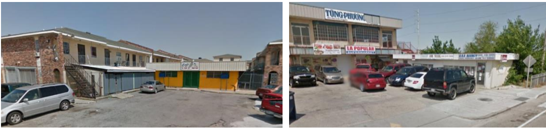
Examples of creative adaptive reuse and infill along the corridor to meet community needs.
