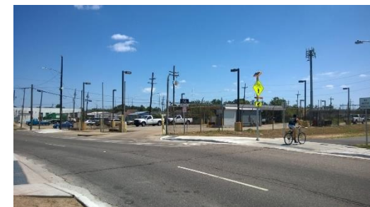
The City's fleet fueling station is located at the intersection of the Lafitte Greenway and Broad St..
