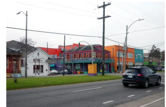
Diverse building types on the corridor
