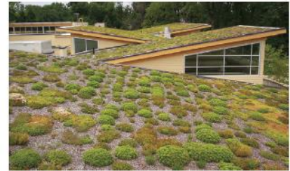
Green Roofs A vegetated roof, planted over a waterproofing membrane, which can help reduce stormwater runoff, lower cooling costs, and provide habitat for wildlife. Photo by Arlington County VA on Flickr/CC
