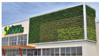
Green Walls A green wall is a vegetated wall, which can provide shade and lower cooling costs.
