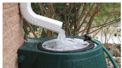
Rain Barrel and Cistern Rain barrels collect and store rainwater for non-potable usage, including landscape irrigation.
