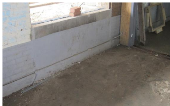
Application of Impermeable Coating
