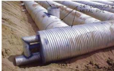
Subsurface Storage Subsurface storage helps detain and store water below ground using vaults, pipe chambers, or plastic structures, to reduce the amount of stormwater entering the drainage system.
