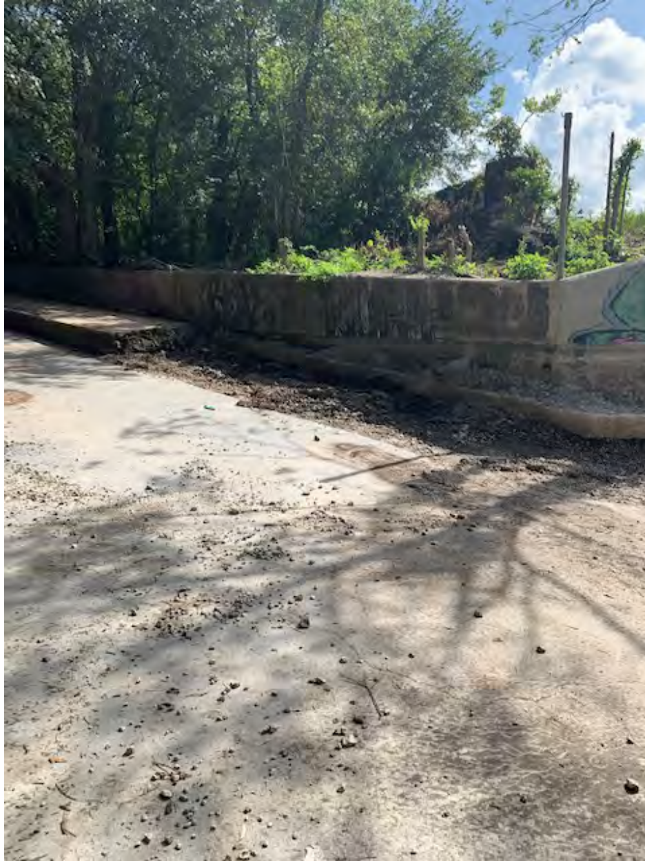
Figure 46: Missing 50'x8' Concrete Walk on East side of Horseshoe Driveway
