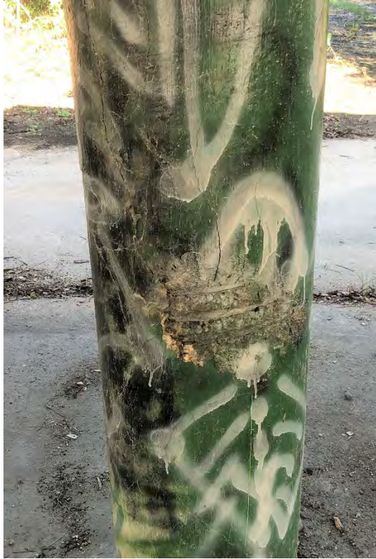
Figure 23: Mid-height spalling at column A3.
