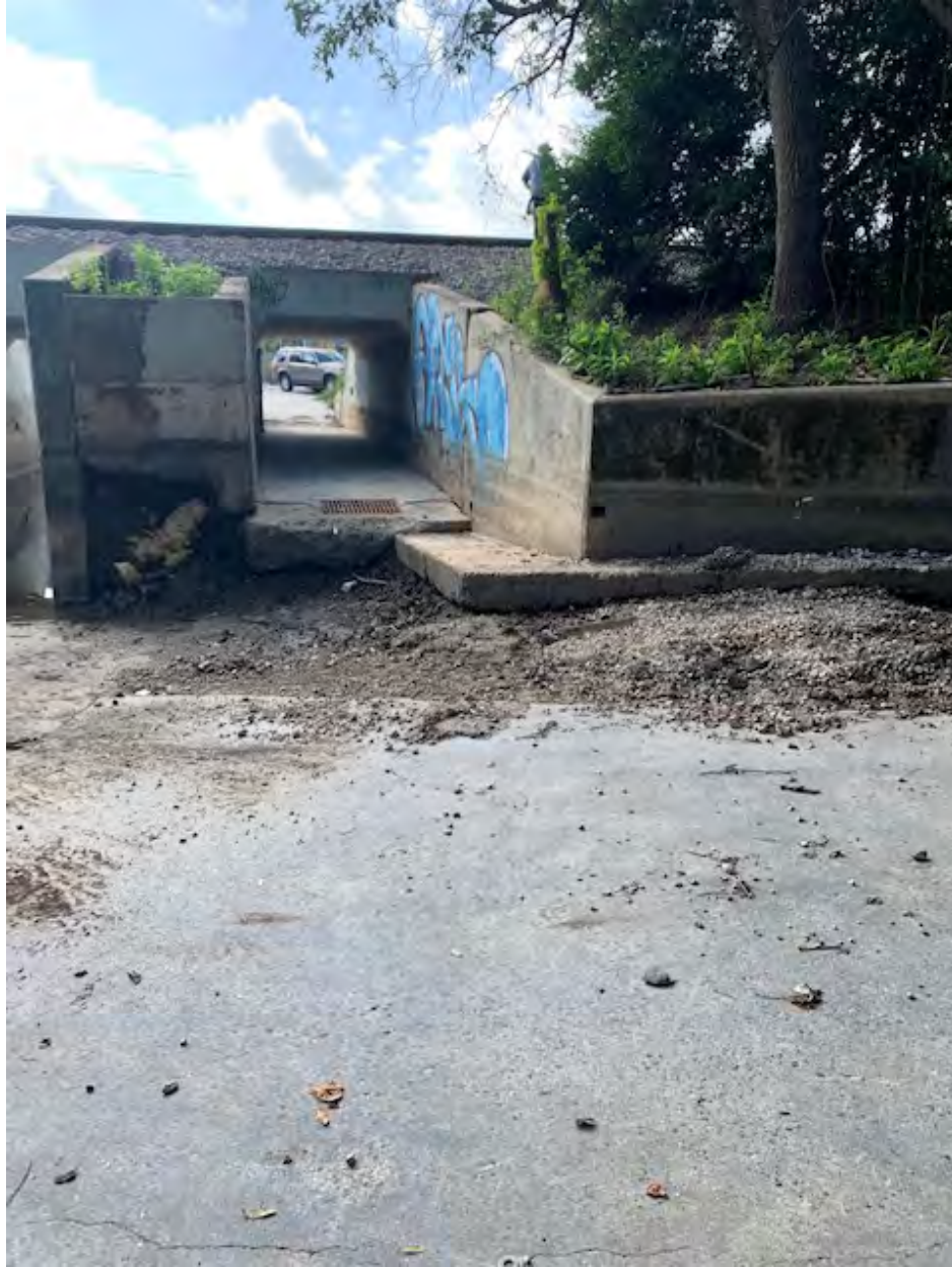
Figure 47: Missing 30'x8' Concrete Walk on West side of Horseshoe Driveway
