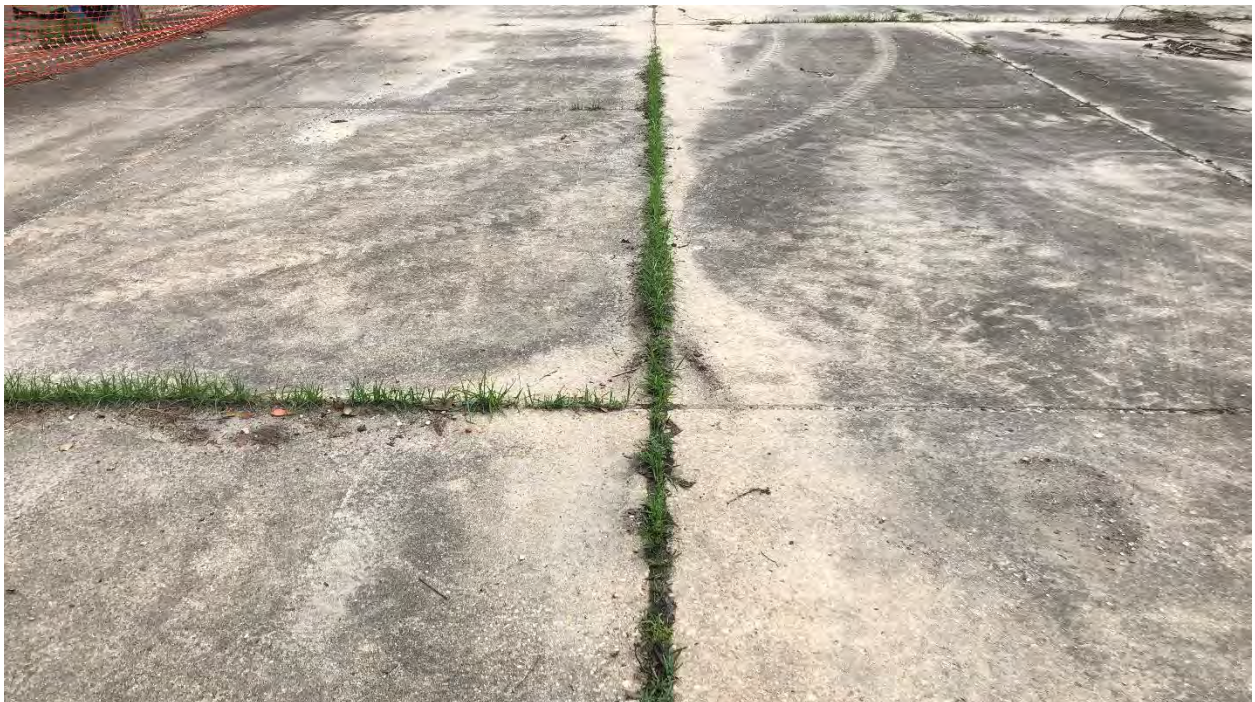
Figure 9: Overgrown joints between concrete panels
