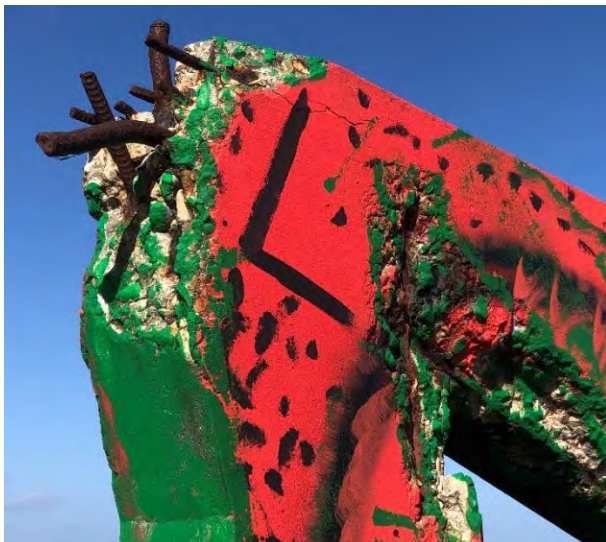
Figure 30: Exposed rebar on where pool canopy connected to support.
