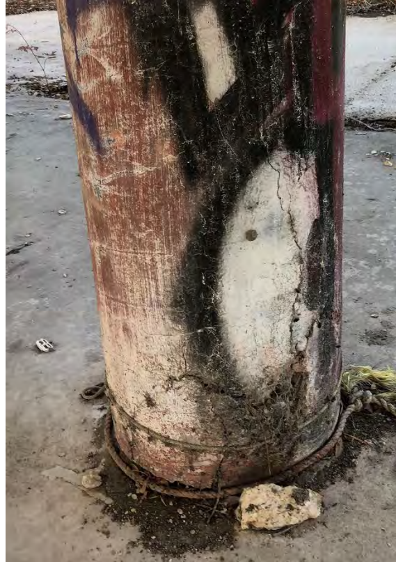
Figure 24: Spalling at bottom of column A5
