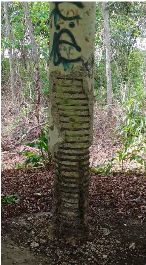
Figure 17: Column A5 showing significant damage before being repaired
