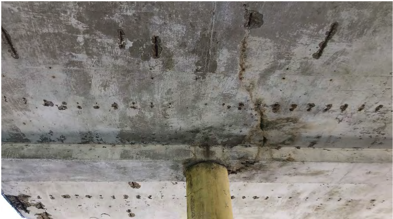
Figure 25: Crack running through roof panel 5 that originates at column A6.
