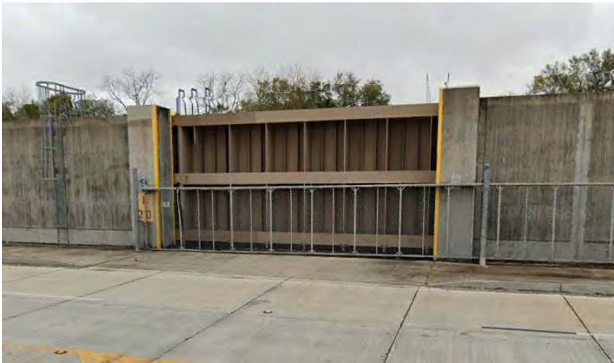
Figure 45: Closed Flood Gate
