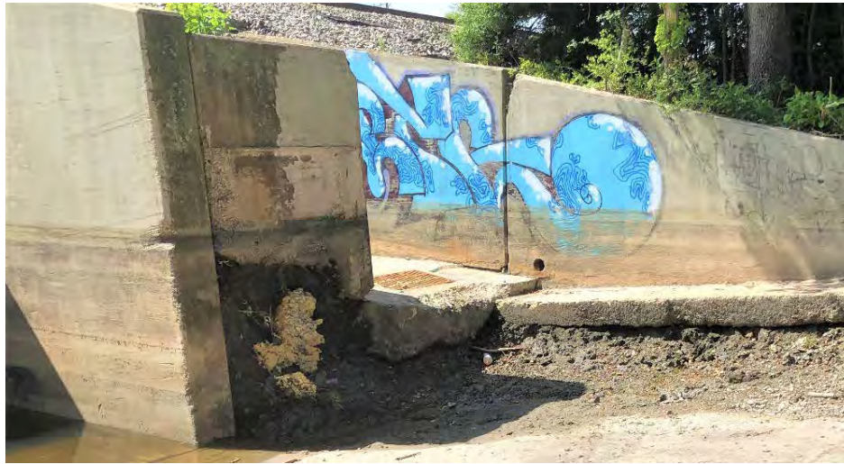
Figure 39: The bottom of the retaining wall is missing, revealing earth beneath the train tracks
