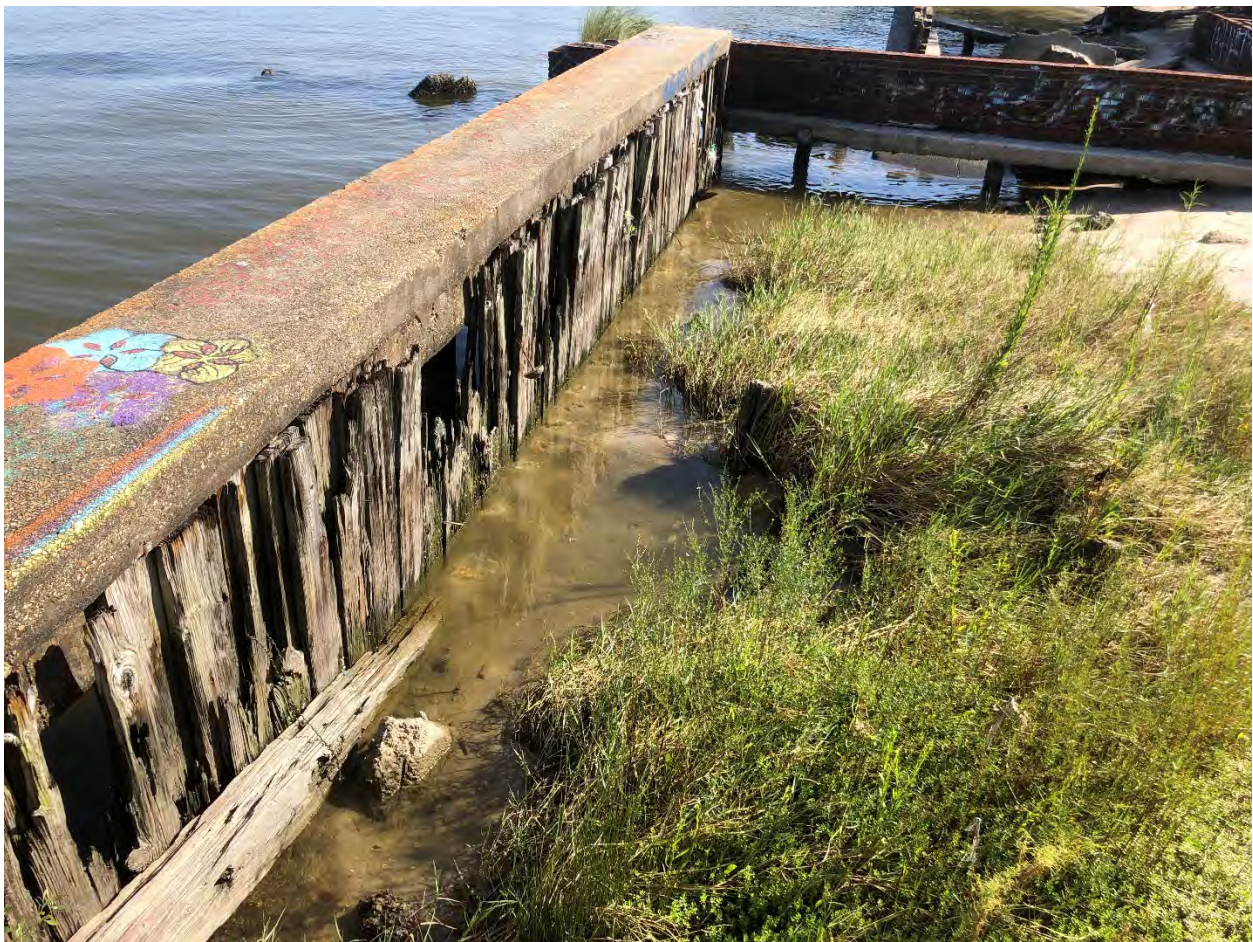
Figure 32: Portion of bulkhead exhibiting damage and erosion of sand
