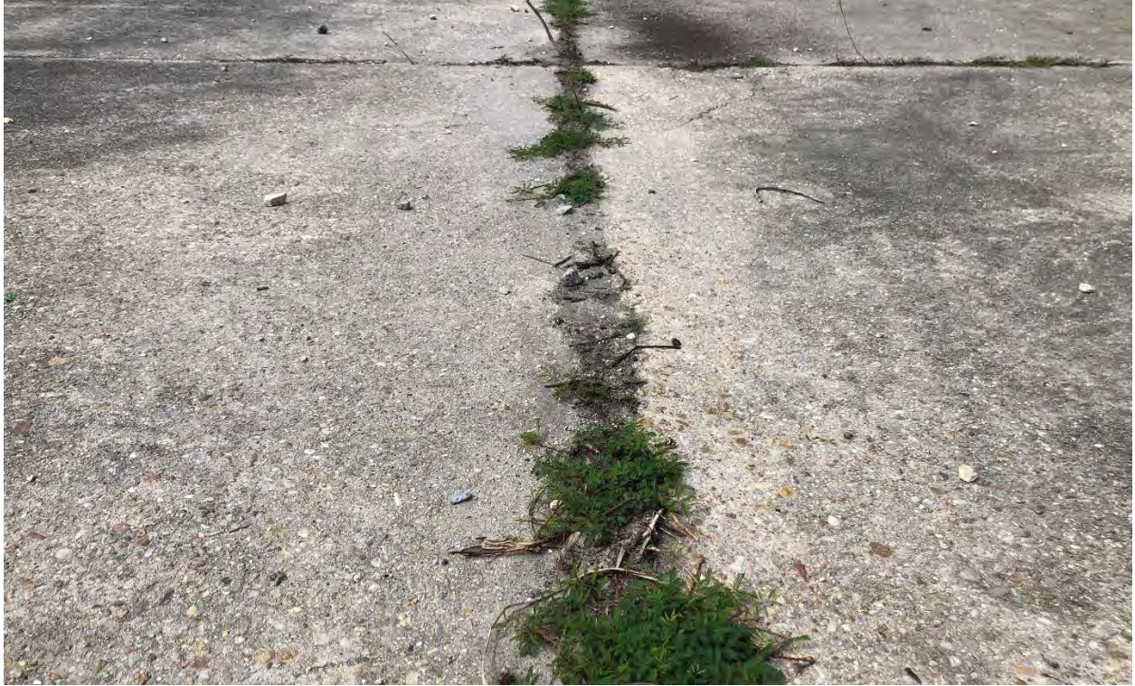
Figure 8: Overgrown joints between concrete panels.
