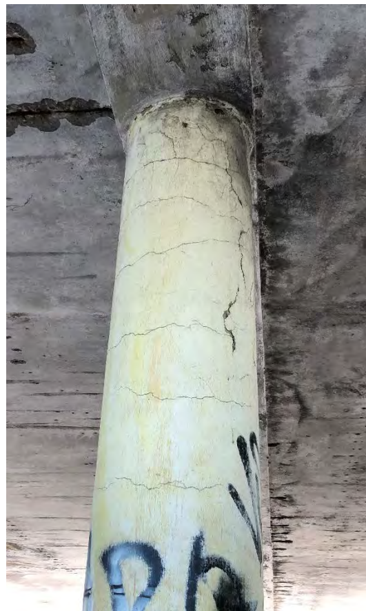
Figure 18: The tops of all columns of the west and east pavilion exhibited this cracking
