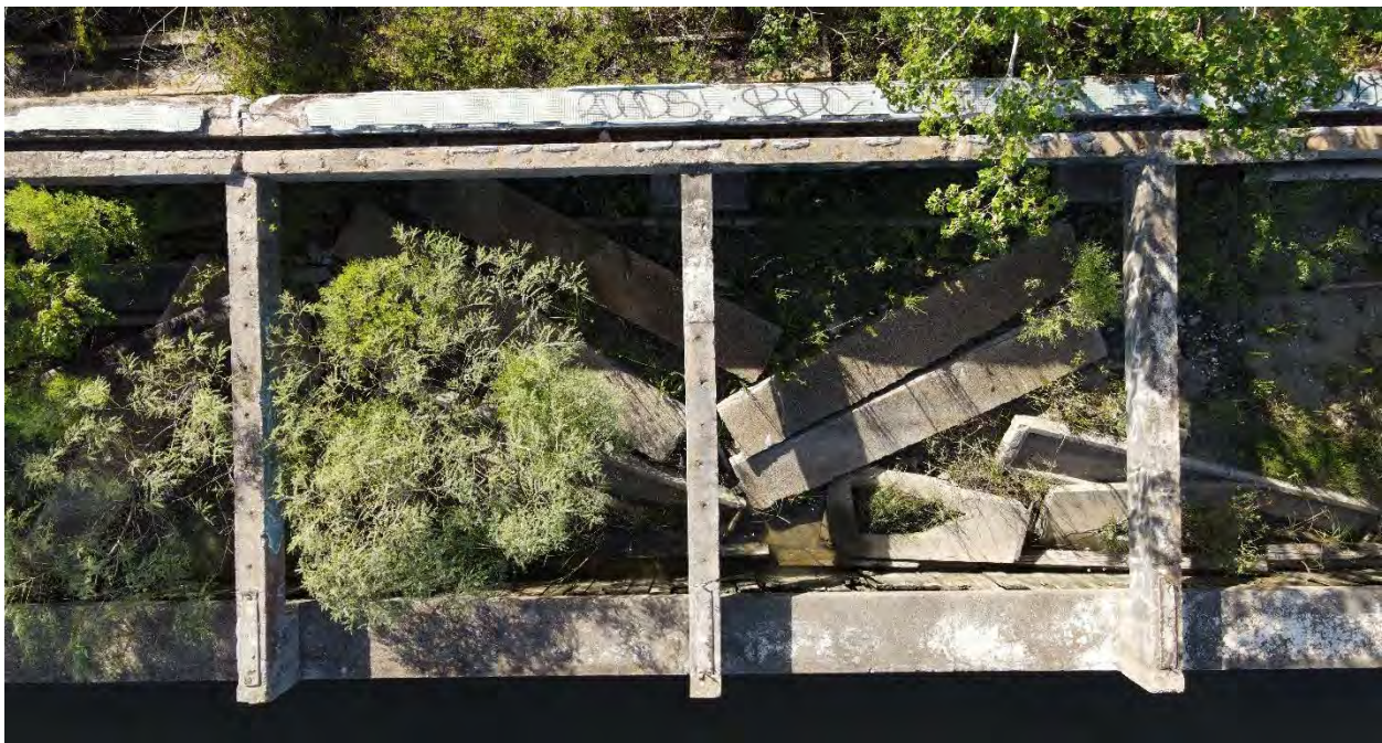
Figure 28: Aerial view of existing deck supports and the washed away concrete decking
