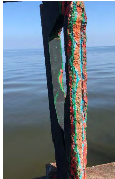
Figure 31: Canopy support with all rebar exposed due to spalling
