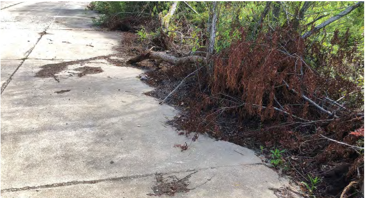
Figure 14: Half of panel cracked and missing in Segment C12.
