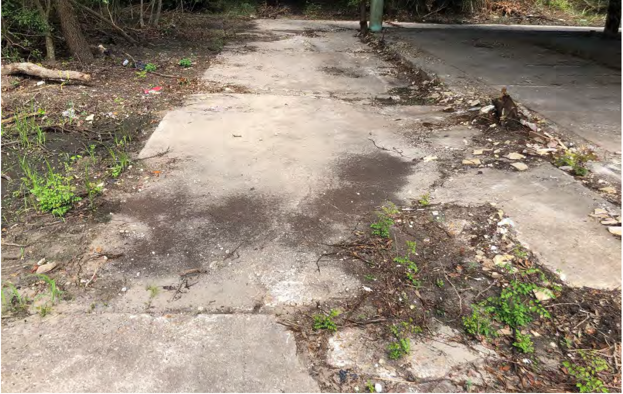
Figure 13: Excessive cracking in Segment A14.
