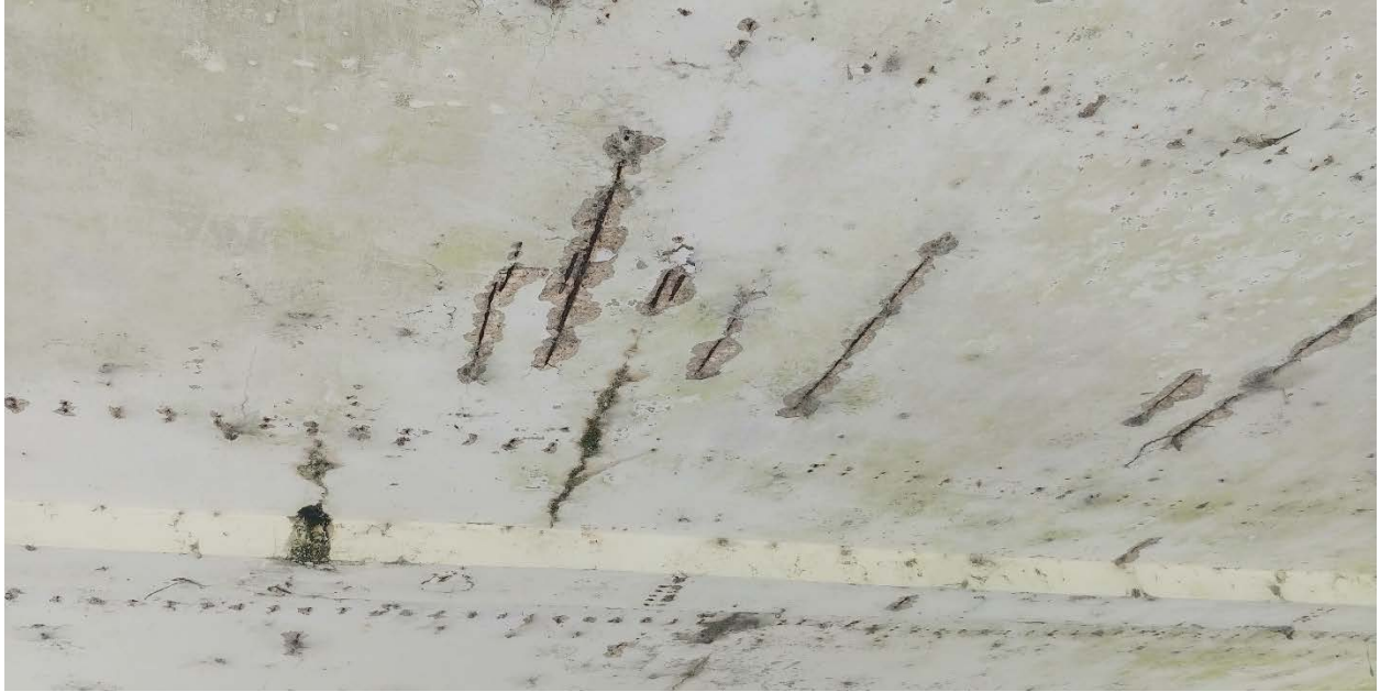
Figure 19: Visible concrete reinforcement caused by incorrect placement of the rebar at the time of the pavilion's construction
