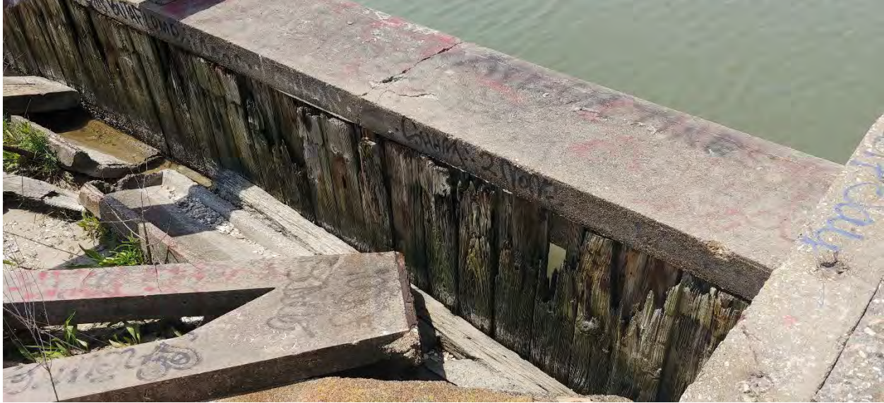
Figure 33: Damaged bulkhead beneath the pool deck supports
