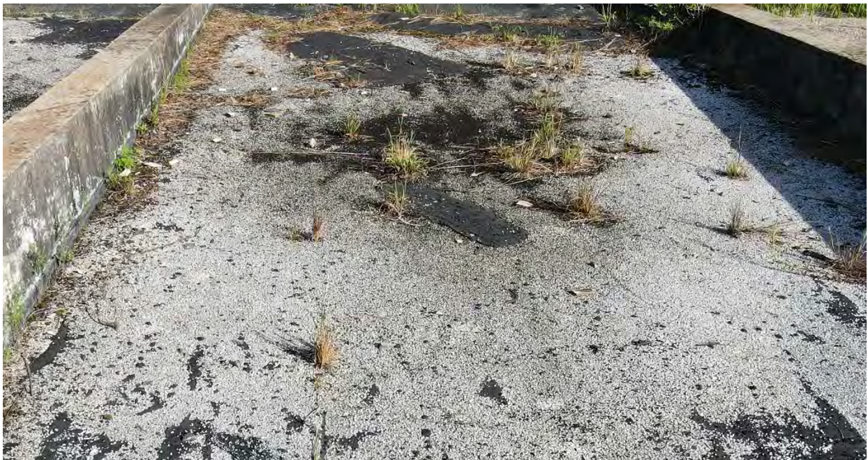
Figure 20: Tar and gravel roof in poor condition
