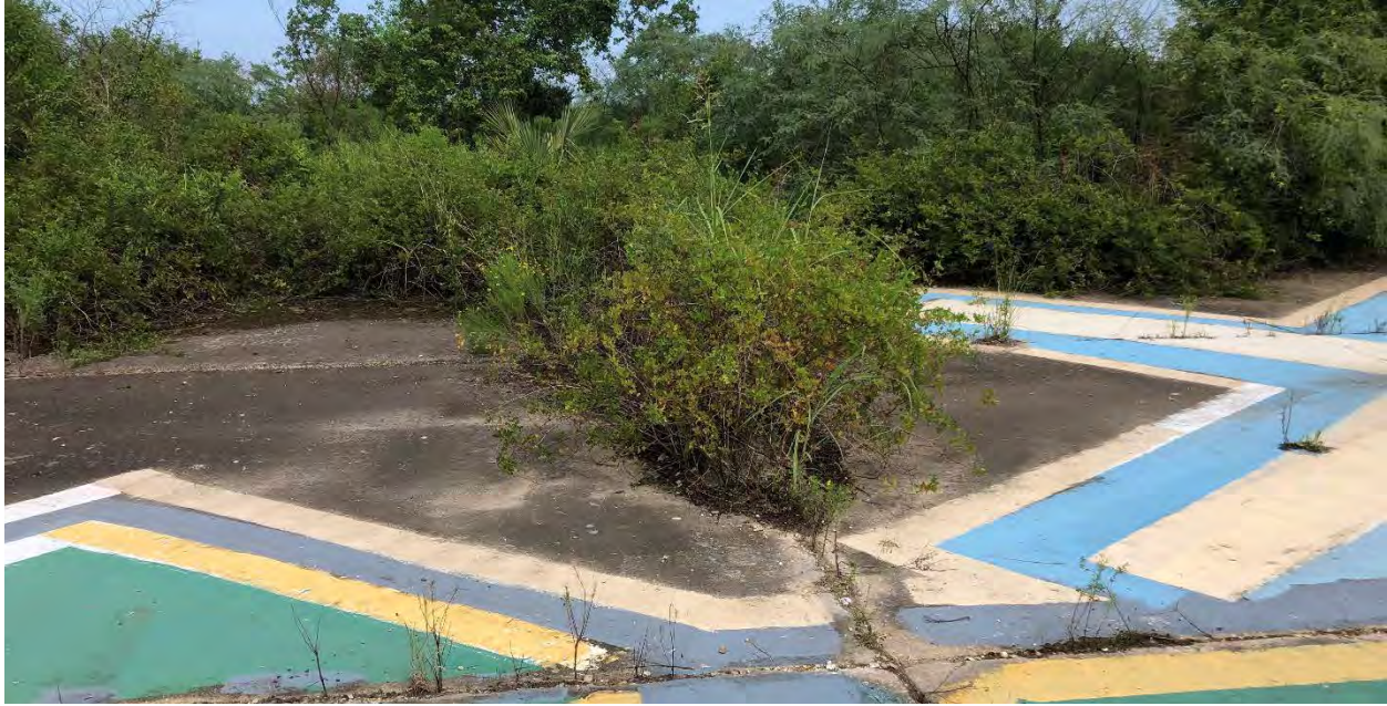
Figure 10: Severe overgrown in concrete joint, likely causing damage to the adjoining panels
