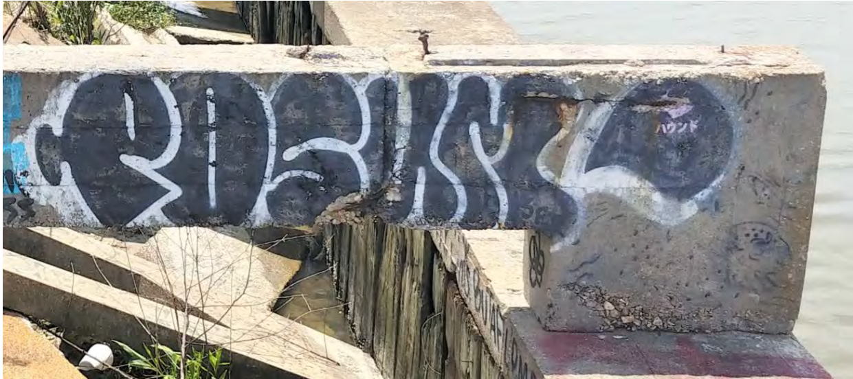
Figure 27: Visual crack through the entire section of the existing deck support
