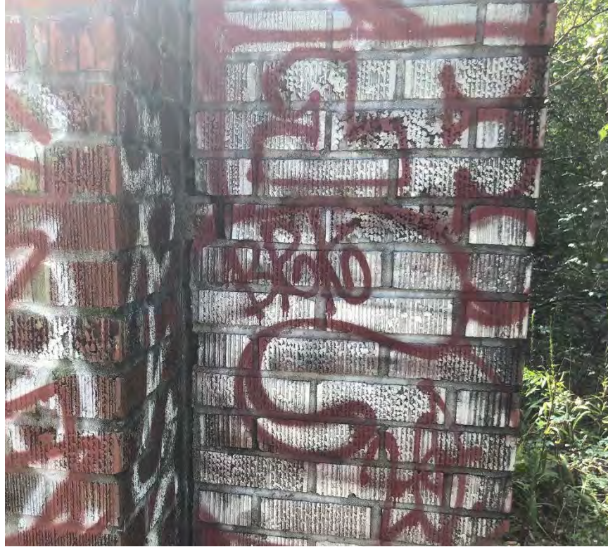
Figure 37: Separation of pilaster from the brick fence
