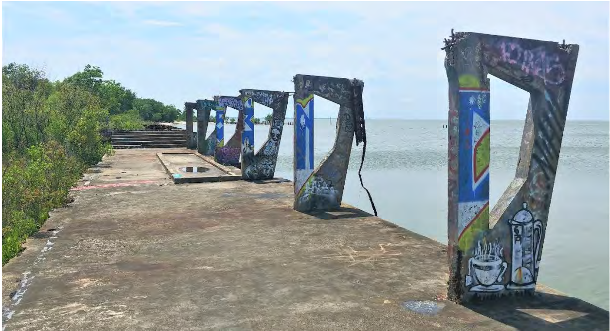
Figure 29: The remaining pool canopy supports remaining on the portion of deck still standing
