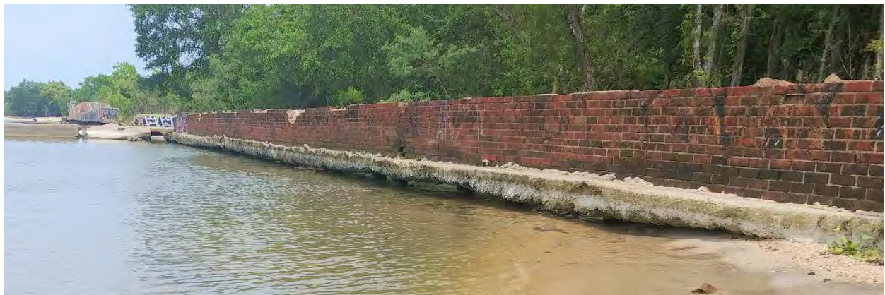
Figure 34: Erosion exposing the underneath of the bulkhead
