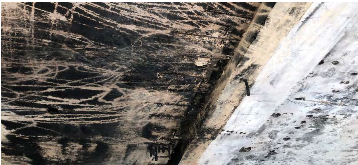
Figure 22: Roof panel 1 with exposed rebar caused by the spalling of concrete under the heat of encampment fires
