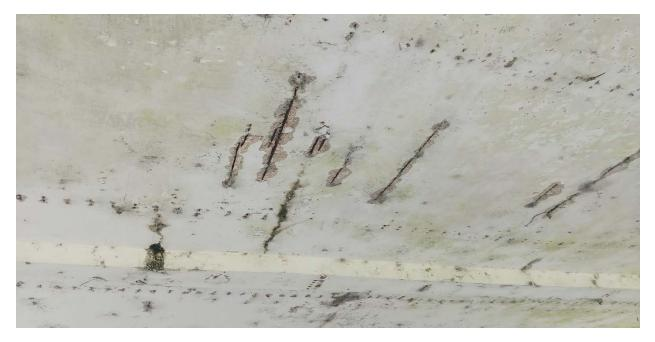
Figure 19: Visible concrete reinforcement caused by incorrect placement of the rebar at the time of the pavilion's construction
