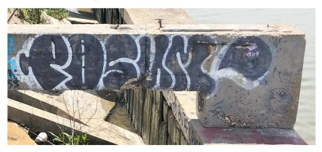
Figure 27: Visual crack through the entire section of the existing deck support
