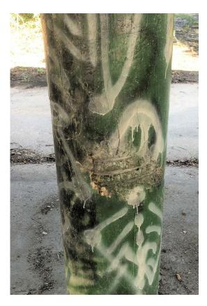
Figure 23: Mid-height spalling at column A3.
