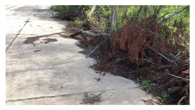
Figure 14: Half of panel cracked and missing in Segment C12.
