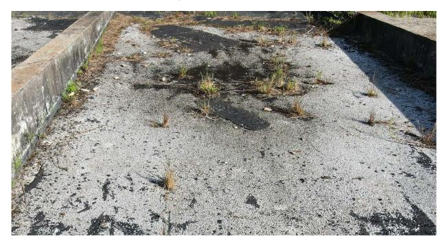
Figure 20: Tar and gravel roof in poor condition
