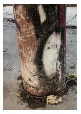
Figure 24: Spalling at bottom of column A5
