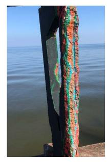
Figure 31: Canopy support with all rebar exposed due to spalling
