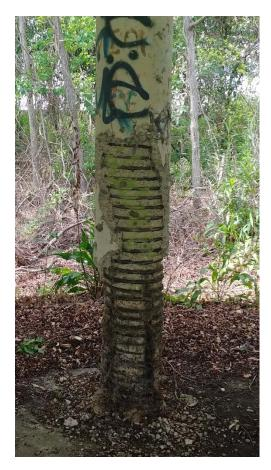
Figure 17: Column A5 showing significant damage before being repaired
