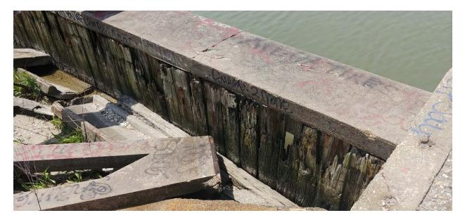
Figure 33: Damaged bulkhead beneath the pool deck supports
