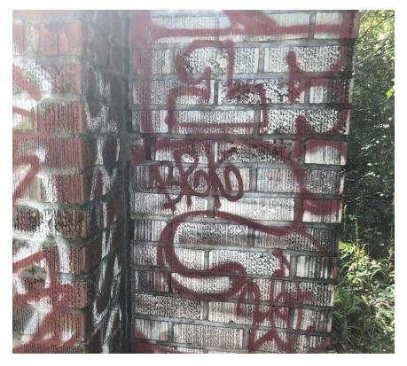
Figure 37: Separation of pilaster from the brick fence
