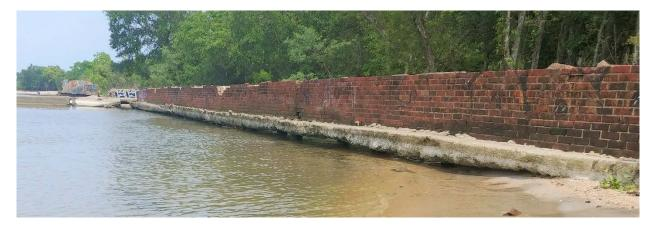
Figure 34: Erosion exposing the underneath of the bulkhead
