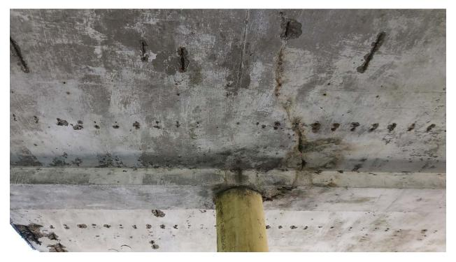
Figure 25: Crack running through roof panel 5 that originates at column A6.
