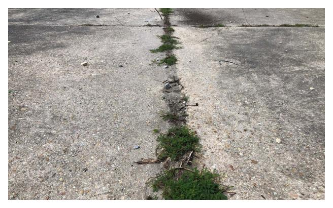
Figure 8: Overgrown joints between concrete panels.
