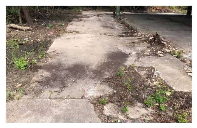
Figure 13: Excessive cracking in Segment A14.
