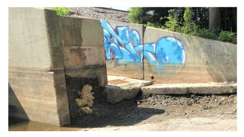
Figure 39: The bottom of the retaining wall is missing, revealing earth beneath the train tracks
