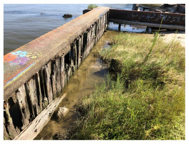
Figure 32: Portion of bulkhead exhibiting damage and erosion of sand
