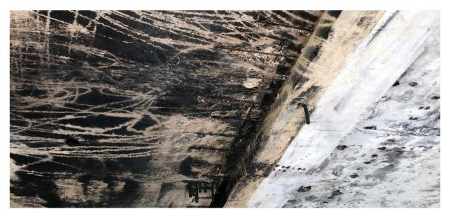
Figure 22: Roof panel 1 with exposed rebar caused by the spalling of concrete under the heat of encampment fires
