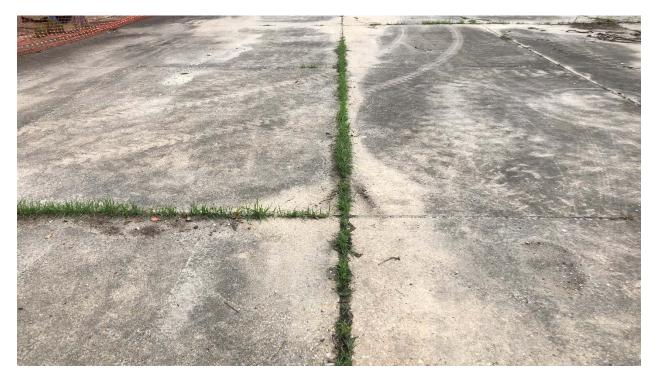
Figure 9: Overgrown joints between concrete panels
