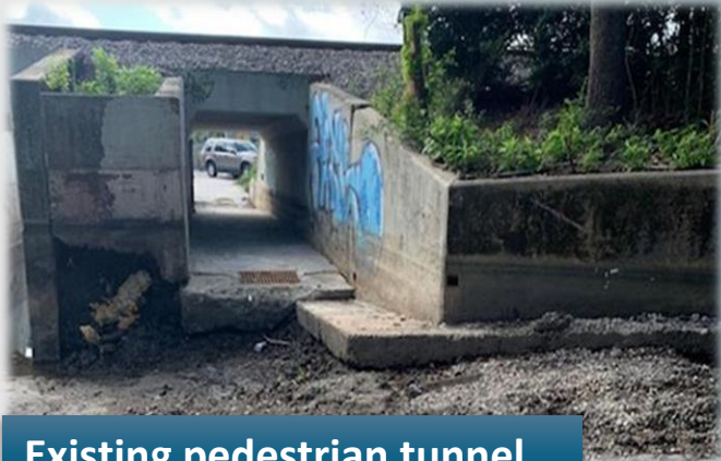
Existing pedestrian tunnel
