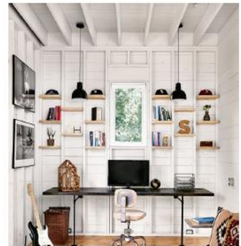
"Perfect" Wall System - Interior Sheathing & studs can become interior wall finish since all insulation is outside of the structure
