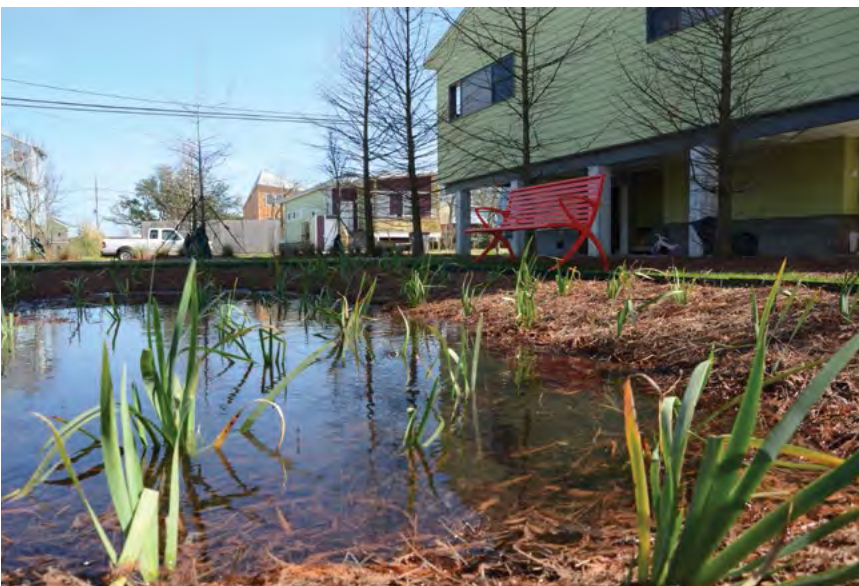
Rain gardens and home elevations, seen here in the Lower Ninth Ward, are examples of ways homeowners can invest in risk reduction.
