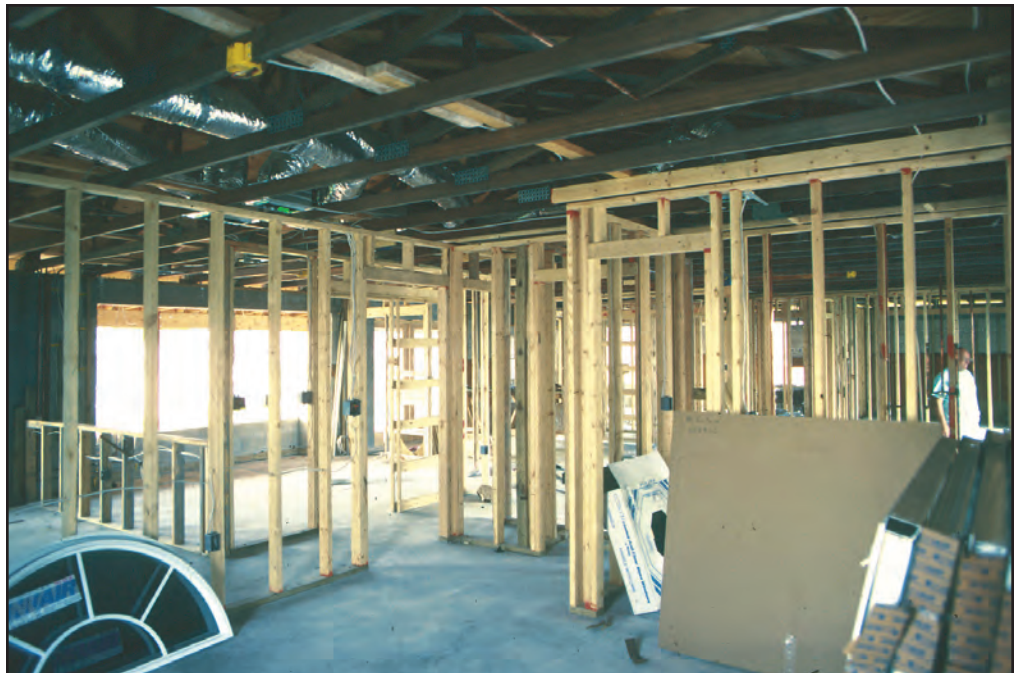
Figure 30 Interior partition walls and utilities are added.
