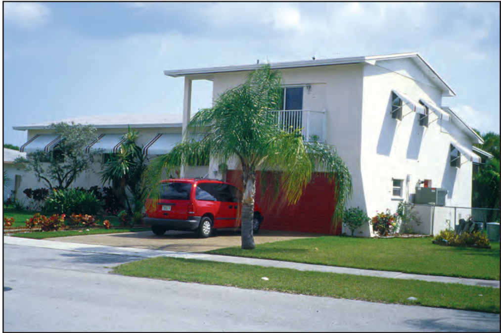
Figure 72 The completed house is compliant with local floodplain management requirements, is more resistant to flood damage, and provides additional living area above the flood level.
