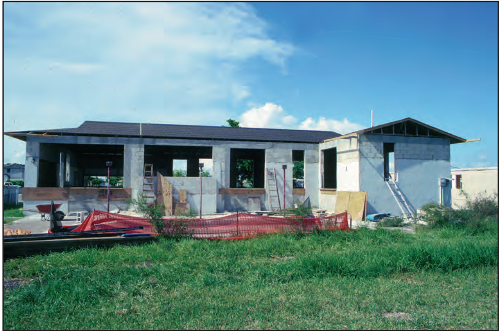
Figure 28 The bottoms of the original window openings are raised with concrete blocks.
