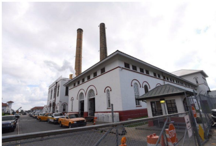
Advocate photo by Matthew Hinton – The Sewerage & Water Board's Carrollton water treatment plant.
