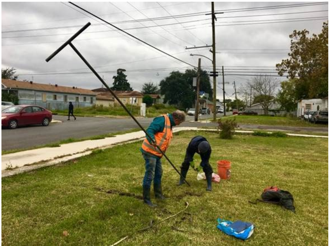
Figure 9.1: Production of shallow borehole
