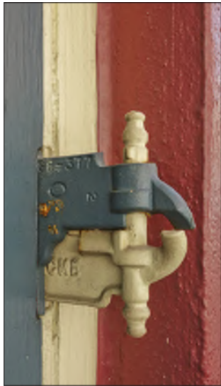
"Acme, Lull & Porter" and "Clark's Tip" hinges hold shutters open and closed, eliminating the need for a shutter dog.
