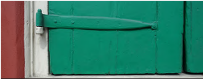
The screwed-in shutters are inoperable and all shutters should be the correct size
