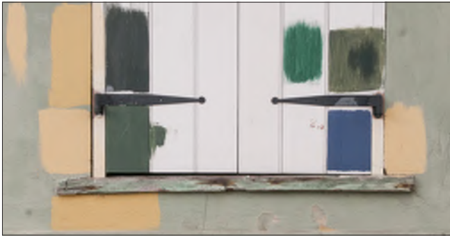
Testing various paint colors on a building provides a better sense of the final appearance than reviewing paint chips.
