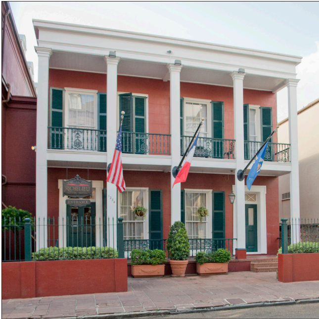
This double Greek Revival townhouse has a two-level, wood-framed gallery extending across the full width of the front façade, supported by rectangular wood posts, known as a double gallery.
