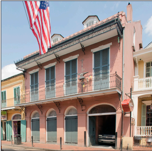
This porte-cochere townhouse includes a carriageway in the right bay, providing access to the rear courtyard. The full-width balcony is accessed by four sets of French doors.
