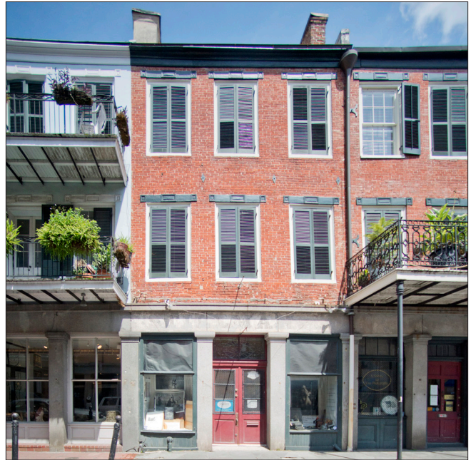
Many of the French Quarter's Greek Revival townhouses include granite piers topped by a granite lintel at the ground floor and a brick or stucco façade above.
