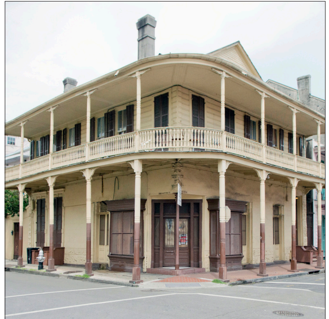
This corner store townhouse includes ground floor commercial space accessed by a corner entry with a residence above. A gallery shelters the sidewalk and provides second floor level outdoor living space.
