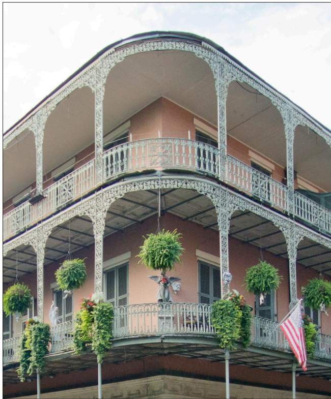
This gallery has delicate and ornate cast iron railings, posts, lintels and brackets that wrap the building's corner.
