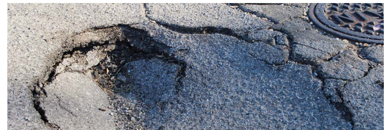
Subsidence-caused Street Damage on Owens Boulevard
