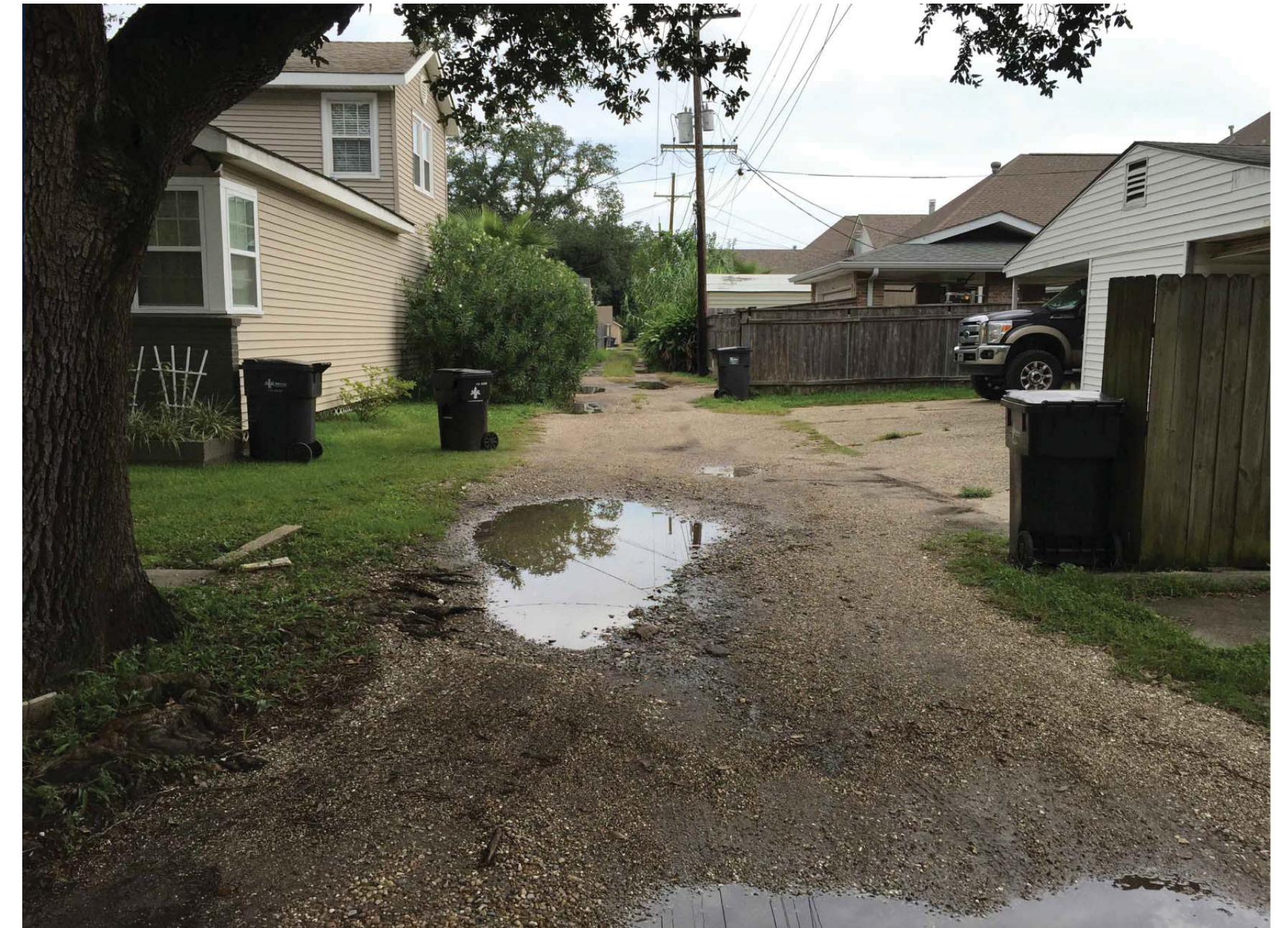
ALLEYWAY, EXISTING CONDITIONS
