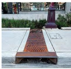
Grate connecting to street bioretention cells
